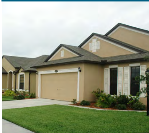
Building America's CARB team worked with Mercedes Homes in east Florida to design homes using cast-in-place concrete walls capable of withstanding wind-blown debris hitting at 200 mph.
