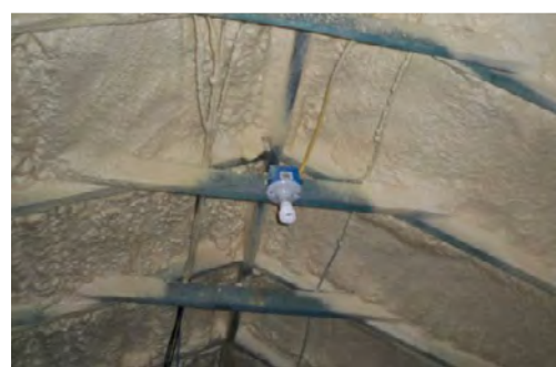
(1) Batt insulation in ceiling. (2) Blown-in insulation. (3) Spray foam. (4) Spray foam applied along the underside of the roof deck to provide a conditioned and non-vented attic space for ducts and air handlers.
