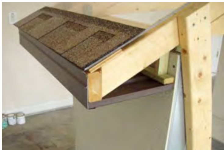
Detail of old soffit showing bottom of assembly is flat with vent perforations facing downward.
