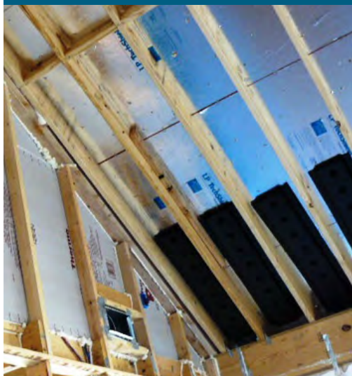
David Weekley Homes uses a radiant barrier product that comes adhered to the underside of the roof sheathing.
