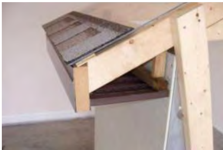
Detail of new soffit design showing extended fascia, providing drip edge.
