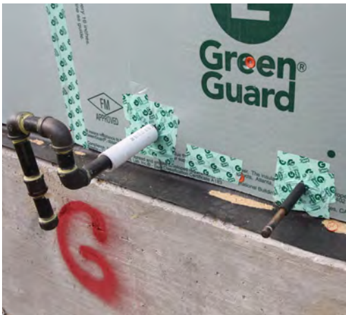
(Top) Attics and walls are insulated with spray foam for superior insulation and air sealing to achieve house leakage of less than 2.5 air changes per hour at 50 Pascals.
