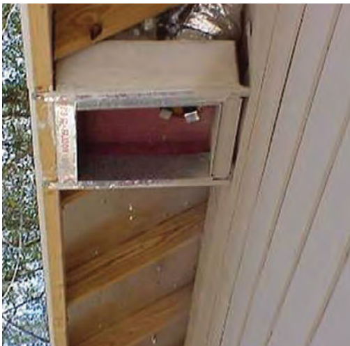
(Top) Tommy Williams Homes uses formaldehyde-free blown fiberglass insulation for R-15 in the walls and R-30 in the attics.
