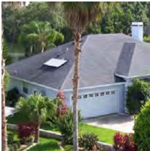
(top) Flat plate collector-style solar water heaters are shown mounted on the roof along with solar photovoltaic panels. (Photo Source: Florida Solar Energy Center)
