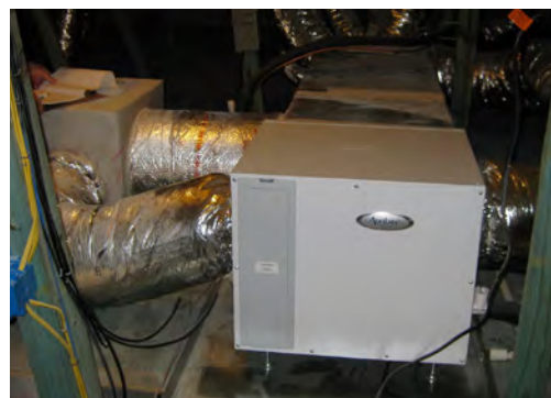
(top) The newest models of air conditioners have efficiencies as high as SEER 20. Follow the manufacturer's recommendations for charging to ensure that high efficiencies are achieved.
