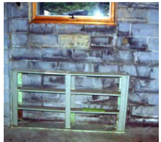
(top) When moisture is trapped inside walls, mold can grow unchecked, causing damage to the walls and health impacts for the occupants. (Photo source: EPA; photo by Terry Brennan)
