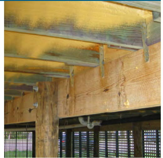
Pier foundations, hurricane strapping, borate- and pressure-treated lumber, and high-density spray foam insulation help homes by Green Coast Enterprises resist the elements in New Orleans.
