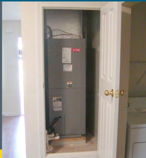
Locating the air handler inside the home reduces energy losses to a hot attic or garage and may lower HVAC installer costs.
