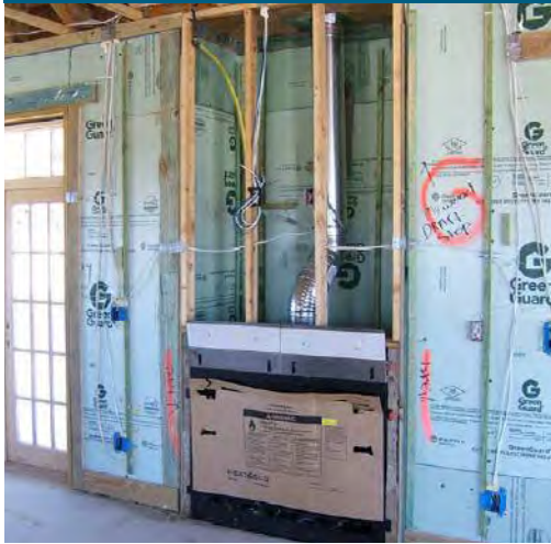
Rigid foam insulates the interior of masonry walls behind the fireplace in this Building America home by Castle and Cooke in Winter Garden, Florida. (Photo Source: BAIHP)
