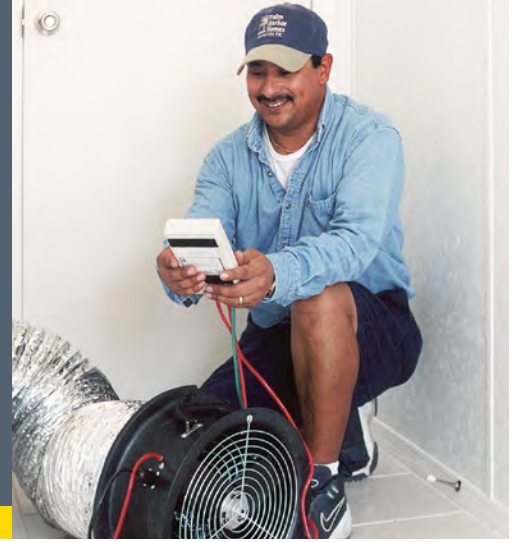
Duct blaster testing confirms that ducts are well sealed ( Photo source: NREL ).
