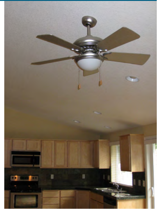
When you add ceiling fans to an air-conditioned room you can drop the thermostat 4 degrees without a noticeable drop in comfort. (Photo Source: PNNL)
