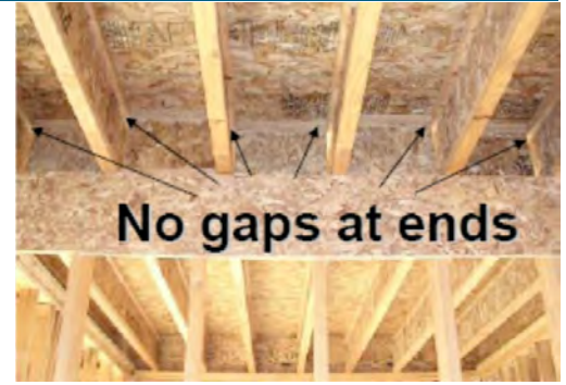
Gaps between garage and conditioned space are properly sealed by carefully cutting and then caulking wood sections to fit between trusses. (Photo Source: EPA 2008)
