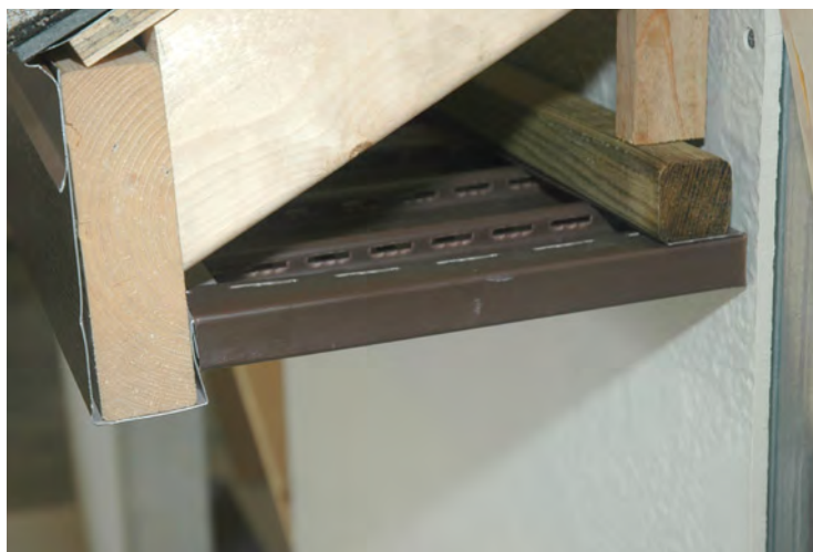
Detail of new soffit design showing fascia and recessed vent perforations.
