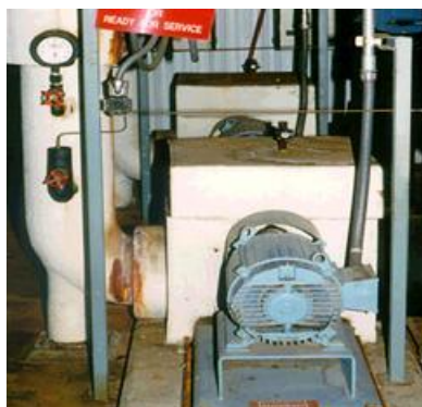
Combined motor & pump efficiency = 59%
