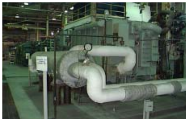
Figure 14: York Prototype Indirect-fired Triple-Effect Chiller
