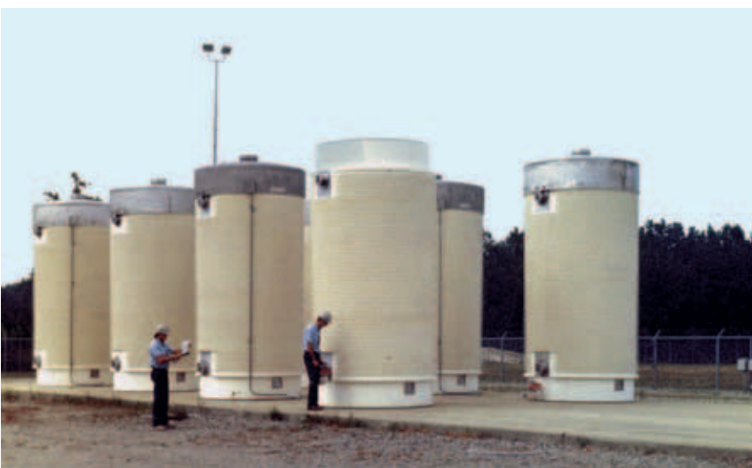
These dry storage casks hold spent nuclear fuel assemblies that have cooled for at least one year.
