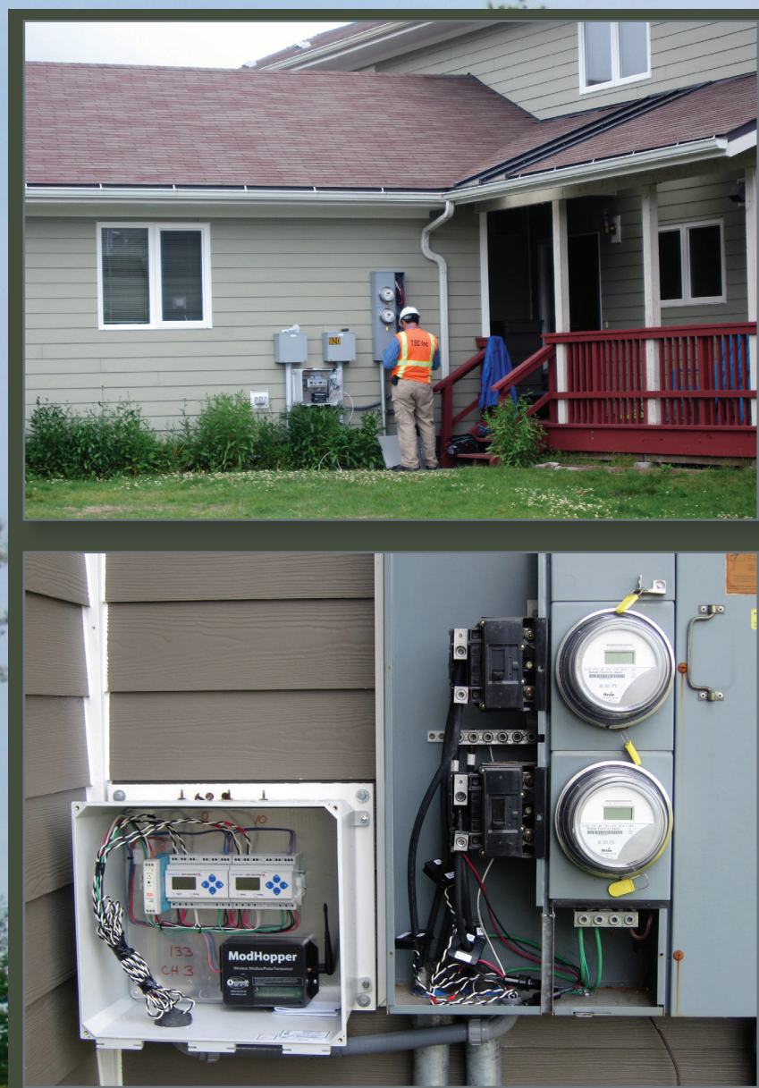
Advanced meters and wireless electricity data transmission provide real time information for Coast Guard facilities.
