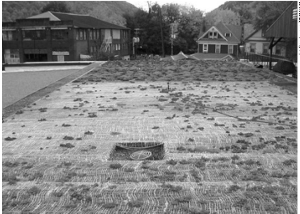
Plants make up a large part of the cost of a green roof. The photo shows establishment using both plant plugs (background) and cuttings (foreground). The plant plugs are forming a dense vegetation cover, whereas the cuttings are developing slowly, leaving most of the soil exposed.
