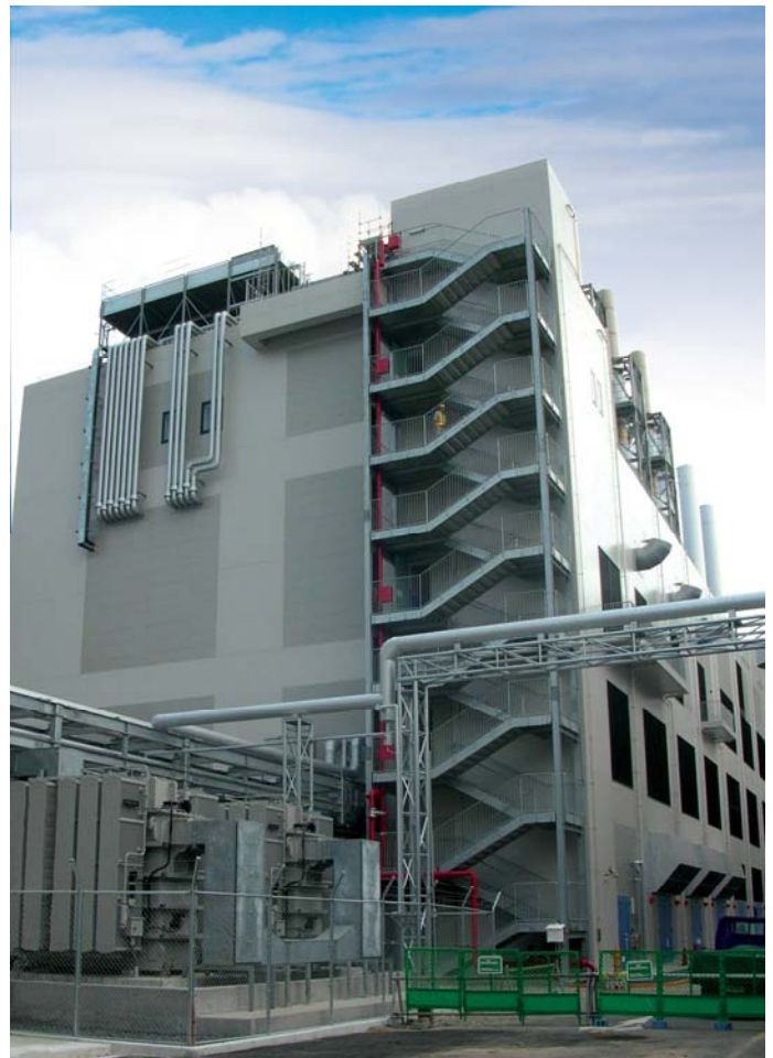
The U.S. Navy Commander Fleet Activities Yokosuka features a 39 megawatt cogeneration plant financed through an ESPC. Photo Courtesy of the Federal Energy Management Program NREL 17253
