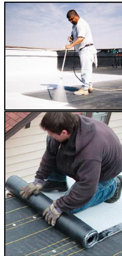
Figure 6: Two Cool Roof Installations
