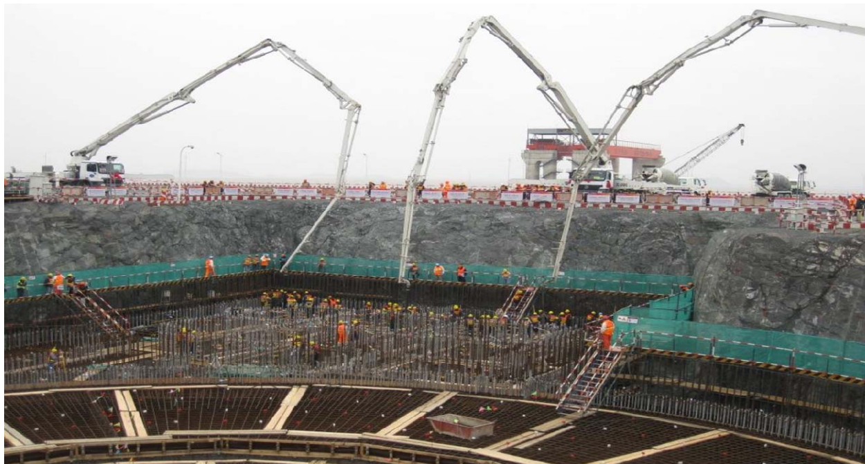
Figure 23. Pouring of First Concrete at Sanmen Unit 1, March 2009
