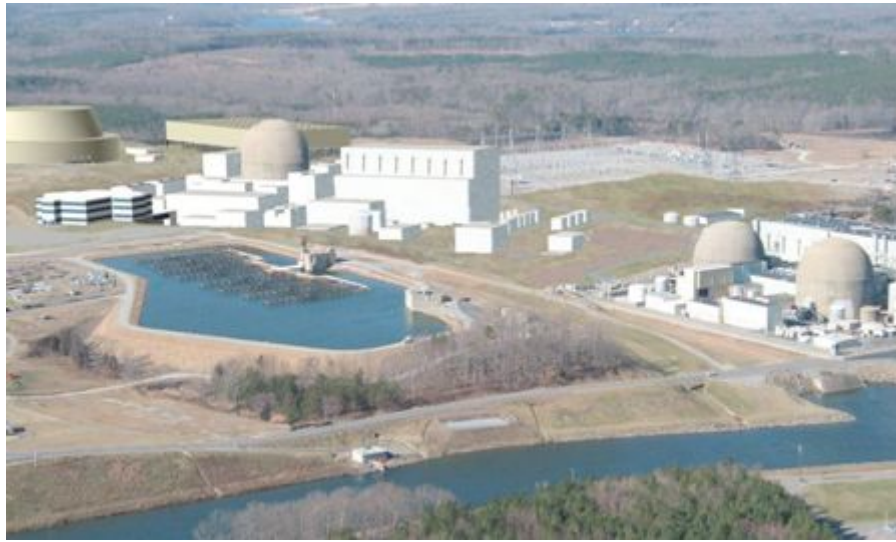
Figure 1: North Anna Station - Unit 3 ESBWR
