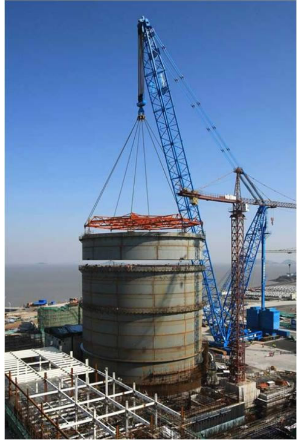
Figure 21. Setting of Containment Vessel Ring Number 4 at Sanmen Unit 1, December 2010
