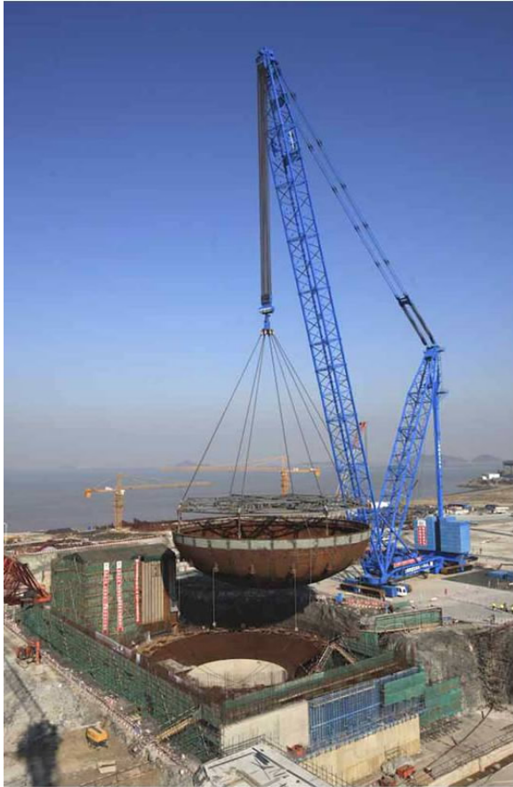
Figure 17. Setting of Containment Vessel Bottom Head at Sanmen Unit 1, December 2009
