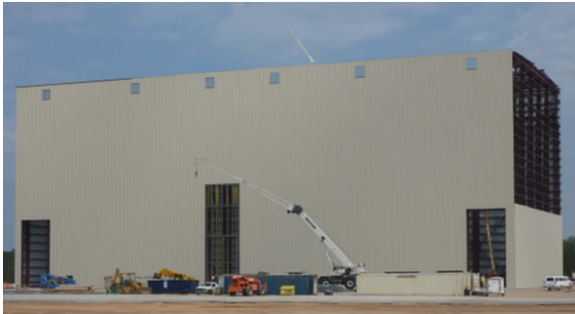
Figure 13. VC Summer Module Assembly Building
