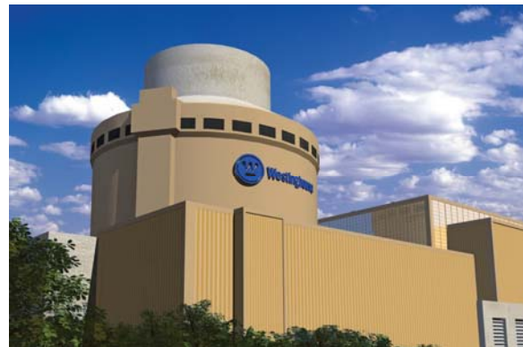
Figure 9. AP1000 Shield Building
