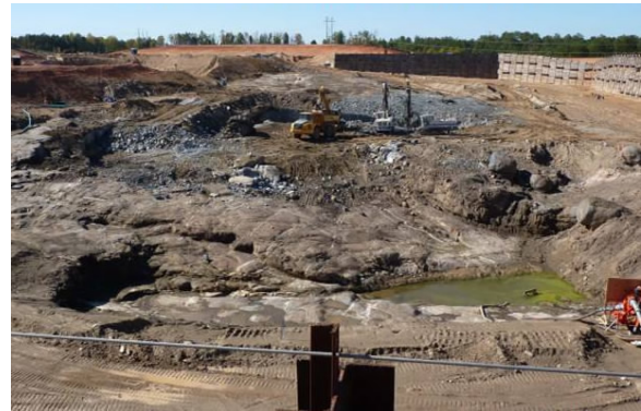
Figure 3. VC Summer Unit 2 Excavation, October 2010
