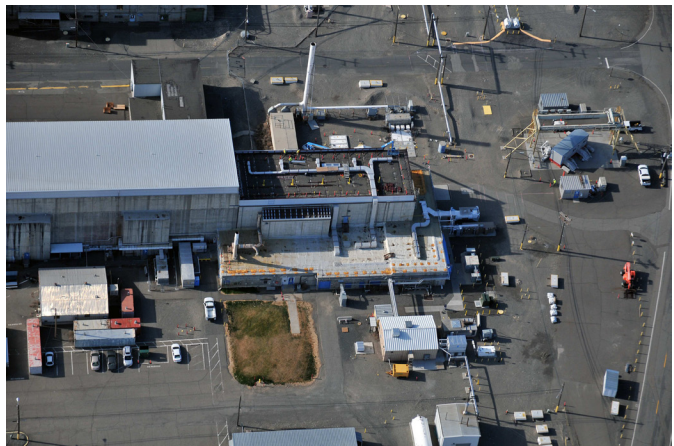
Interior and Aerial Views of the Hanford Site Waste Encapsulation Storage Facility
