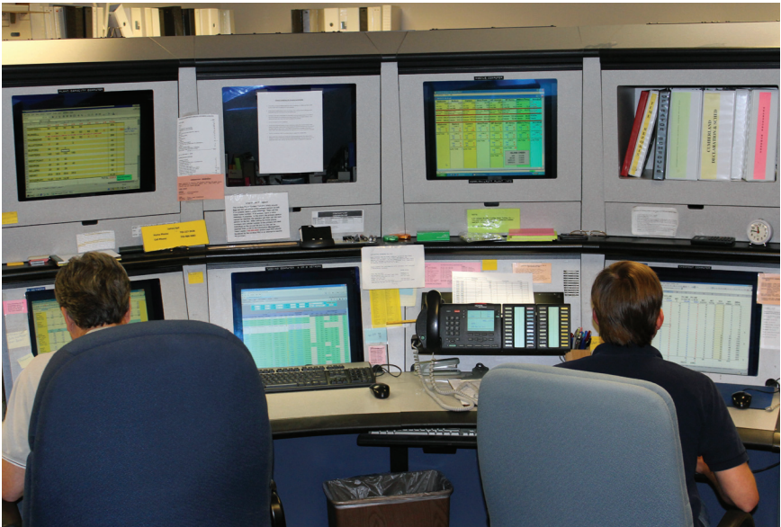
Computer terminals in the new operations center.
