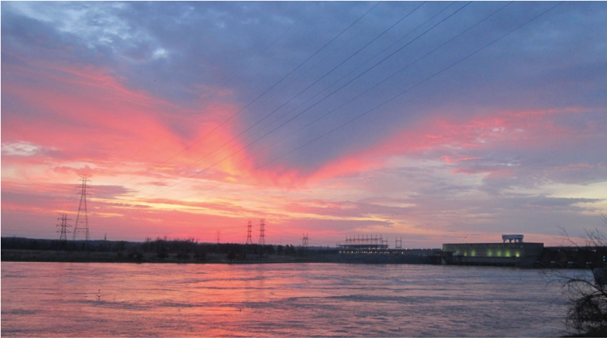
SEPA has no transmission assets. The Corps owns the switchyards and ancillary equipment at the hydro projects, and the external transmission lines are owned by private utilities (Corps photo).
