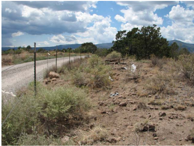
Figure 1. LA 4601B, before wattle installation.
