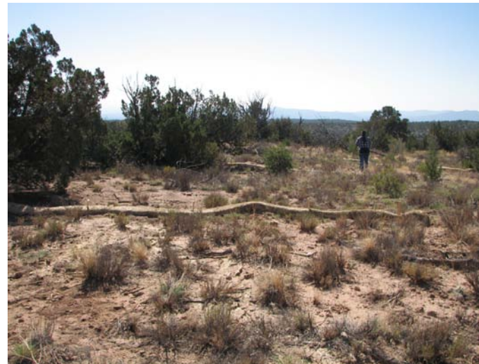
Figure 4. LA 4602A, after wattle installation.
