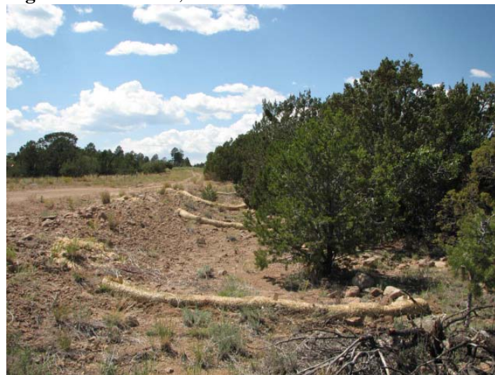
Figure 8. LA 4697, after wattle installation.
