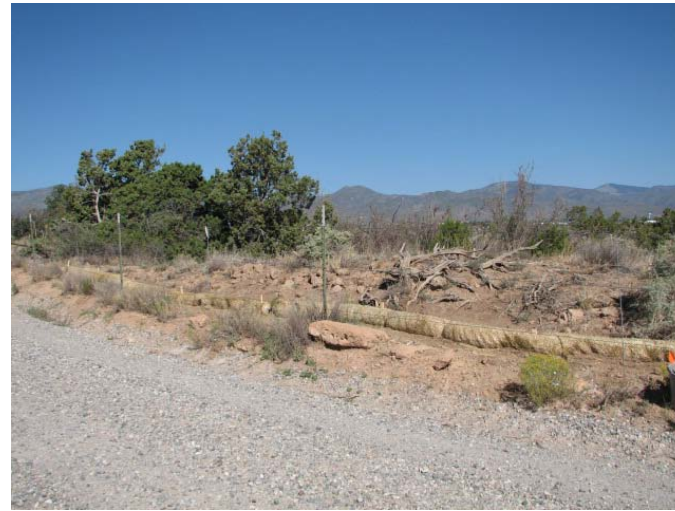
Figure 2. LA 4601B, after wattle installation.
