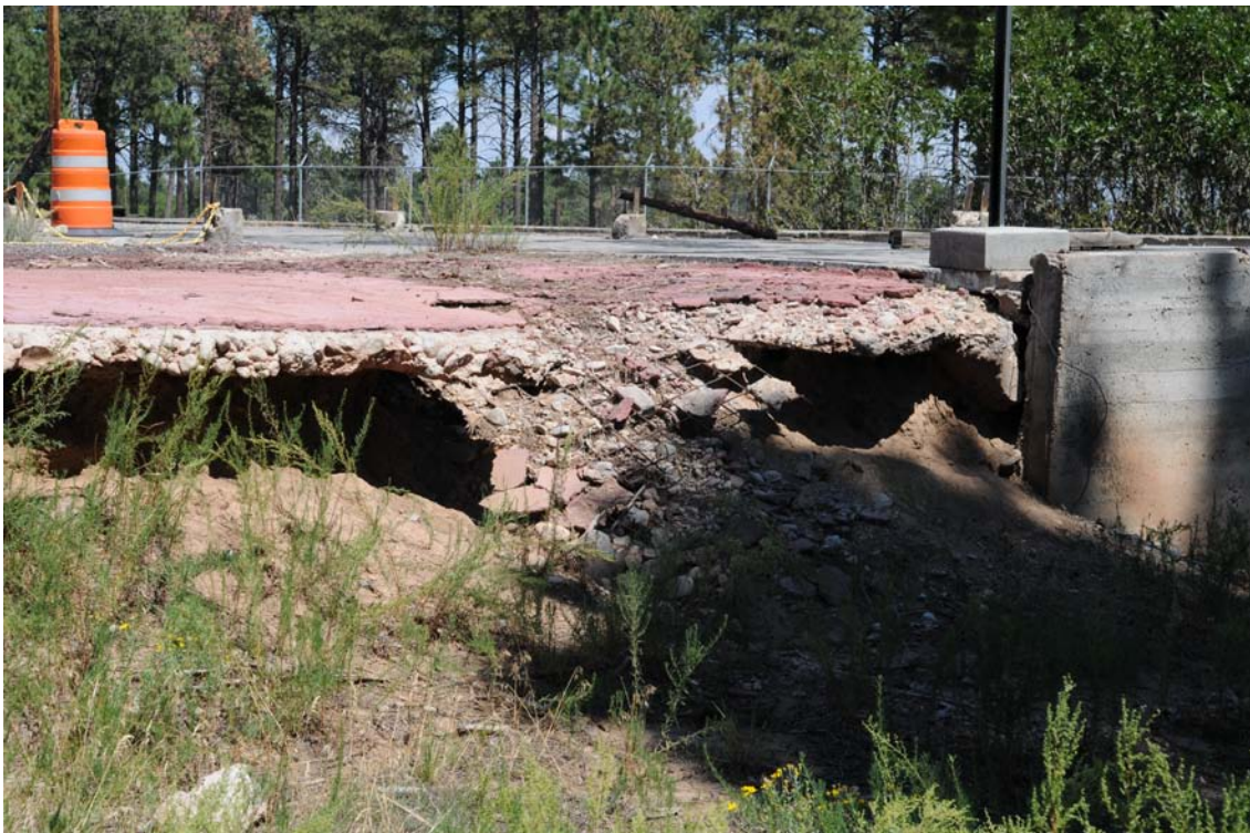
Figure 11 (top) and 12 (bottom). Burned and deteriorating concrete pads (former building locations) at V-Site (2012).
