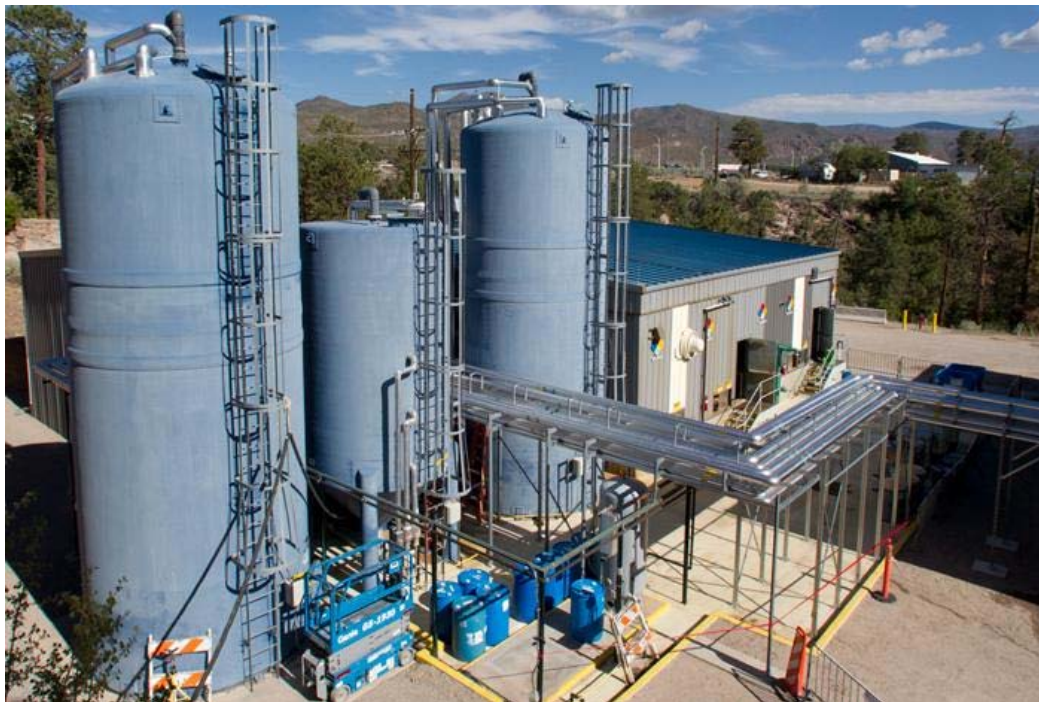
New expansion of the Sanitary Effluent Reclamation Facility (SERF-E).
