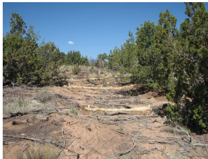
Figure 6. LA 4602B, after wattle installation.
