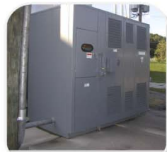
750kVA/2.4kV/480V transformer for rotating based test system and 100kW microturbine on ckt. 4.
