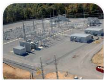
ORNL substation drops voltage from 161 to 13.8kV.
