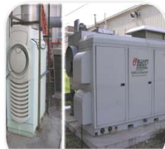
30 kW and 100kW rated microturbines on ckt. 4.
