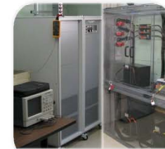
Inverter-based test system with programmable dc power supply on ckt. 2.
