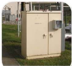
750kVA/2.4kV/480V transformer for inverter test system, load banks, and motors on ckt. 2.
