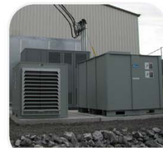
500kW resistive ( \pm 1kW steps) and 375kVar reactive ( \pm 3.75kVar steps) load banks on ckt. 2.
