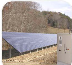
50 kW solar photovoltaic (PV) array across from DECC Lab and PV inverter on ckt. 4.
