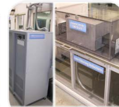
Larger inverter-based test system with programmable DC power supply on ckt. 2.
