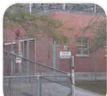
3000 substation drops voltage from 13.8 to 2.4kV to feed DECC Lab through ckt. 2 and 4.
