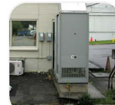
500kW resistive ( \pm 1kW steps) load bank with individual phase control on ckt. 2.
