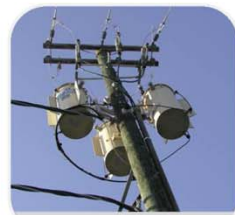
300kVA/2.4kV/480V transformer for PV inverter and 30kW microturbine on ckt. 4.
