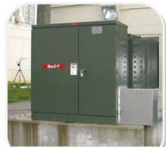
1500kVA/2.4kV/480V transformer for larger inverter-based test system on ckt. 2.
