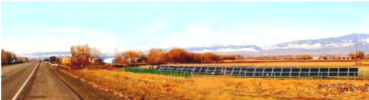
Figure 3-3. Current view of solar panels at the City of Ellensburg's Renewable Energy Park along the eastern side of I-90.
