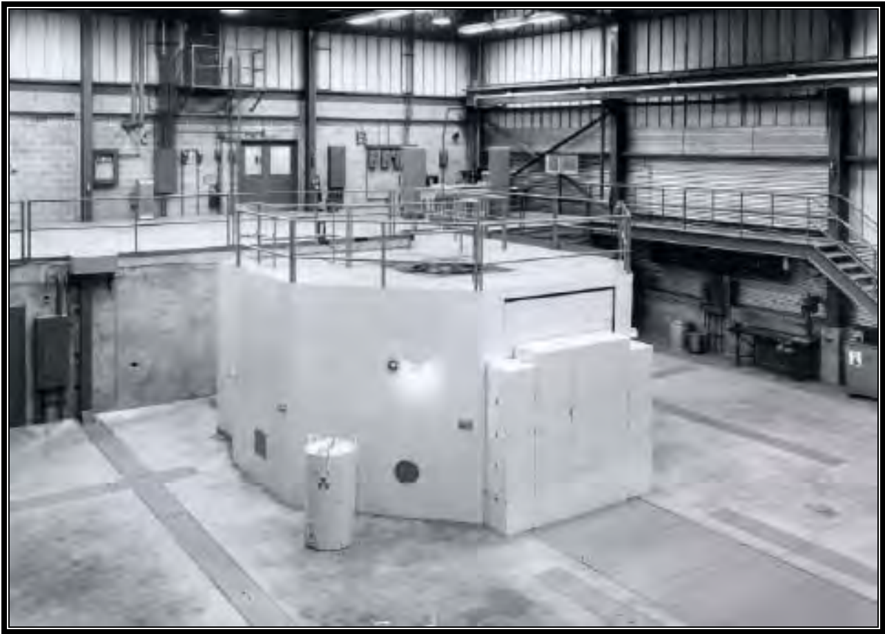
Figure 1-1. Juggernaut Reactor, inside Building 335
