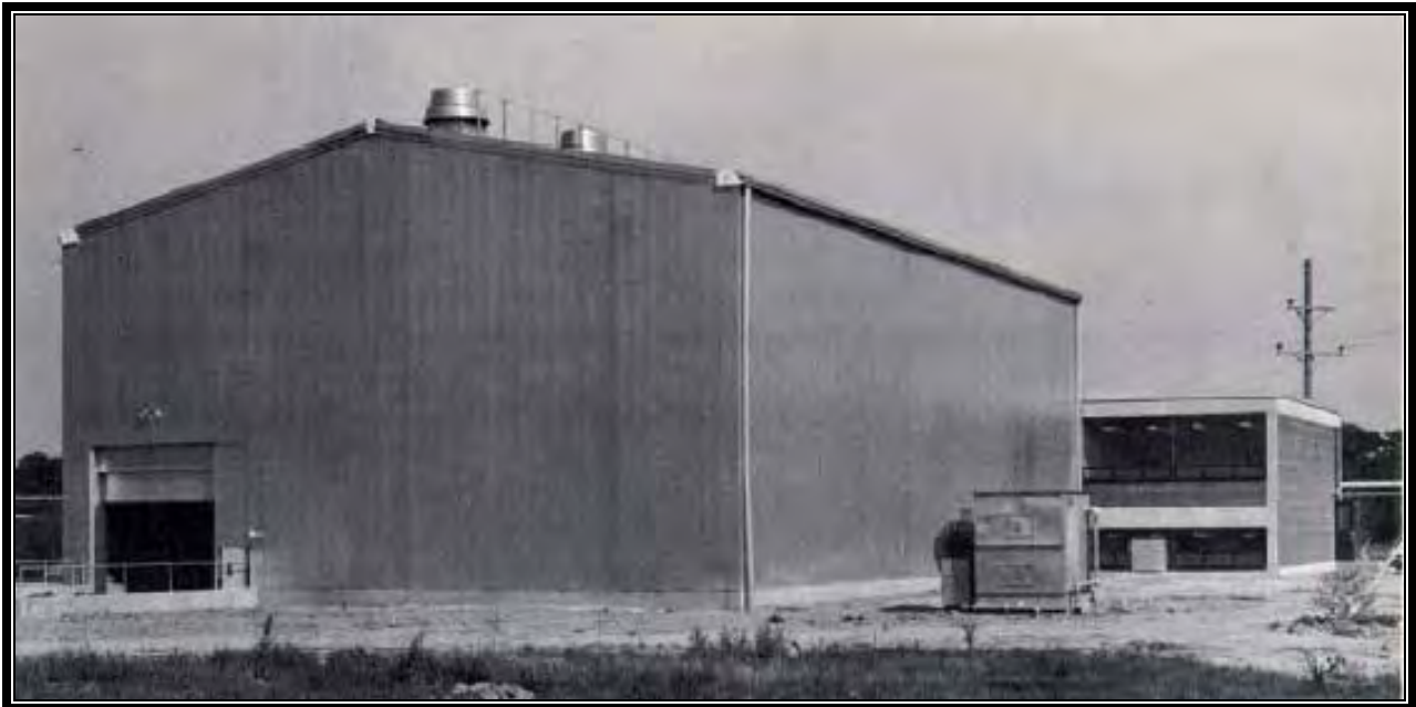
Figure 1-4. Building 335, rear view showing reactor building and cooling tower
