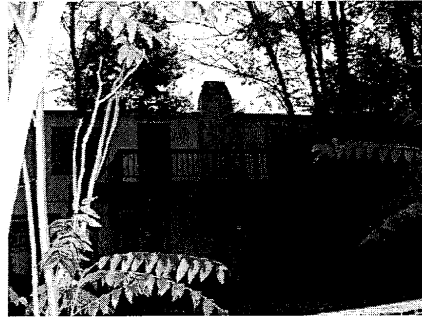
Figure 12. Undamaged chimney of the house (Photo: Goel).
