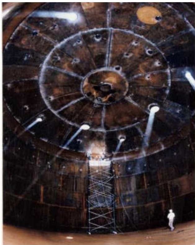
Inside Double-Shell Tank
