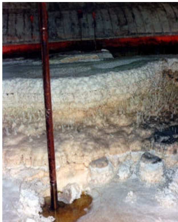
Waste Inside a Single-Shell Tank in the B Tank Farm at the Hanford Site
