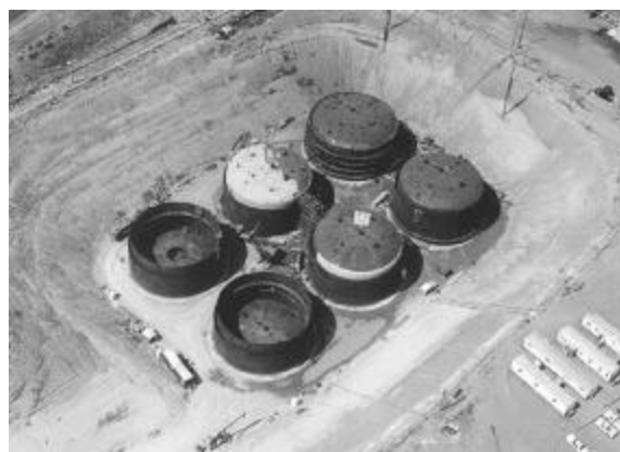
Hanford Site Tank Farm During Construction
