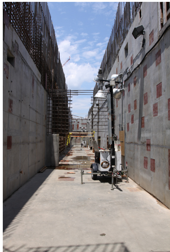
Construction Activities at MOX
