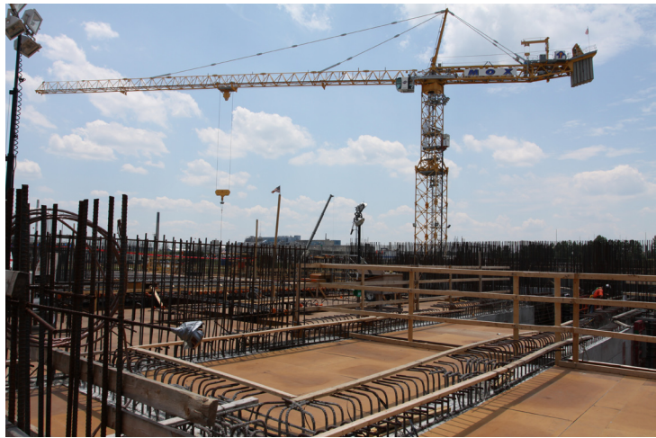
Construction Activities at MOX
