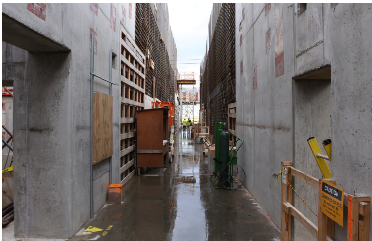
Construction Activities at MOX
