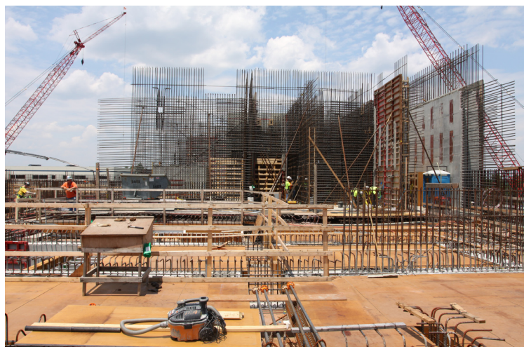
Construction Activities at MOX
