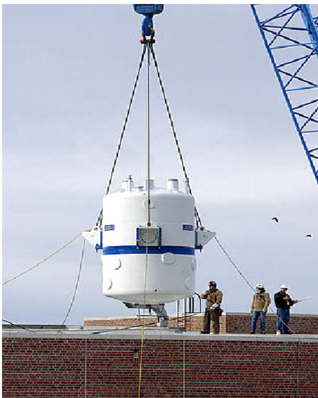
Installation of 16-ton Superconducting Magnet at EMSL
