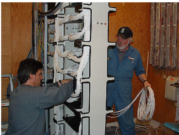
New LAN Installation
