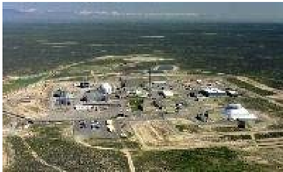
Aerial View of ANL-W
