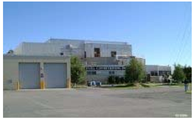
Fuel Conditioning Facility
