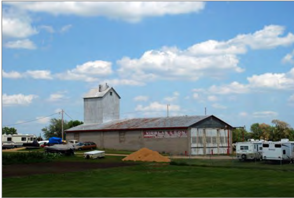
Field No. 52, Virblas and Son Concrete Supply, facing NE
