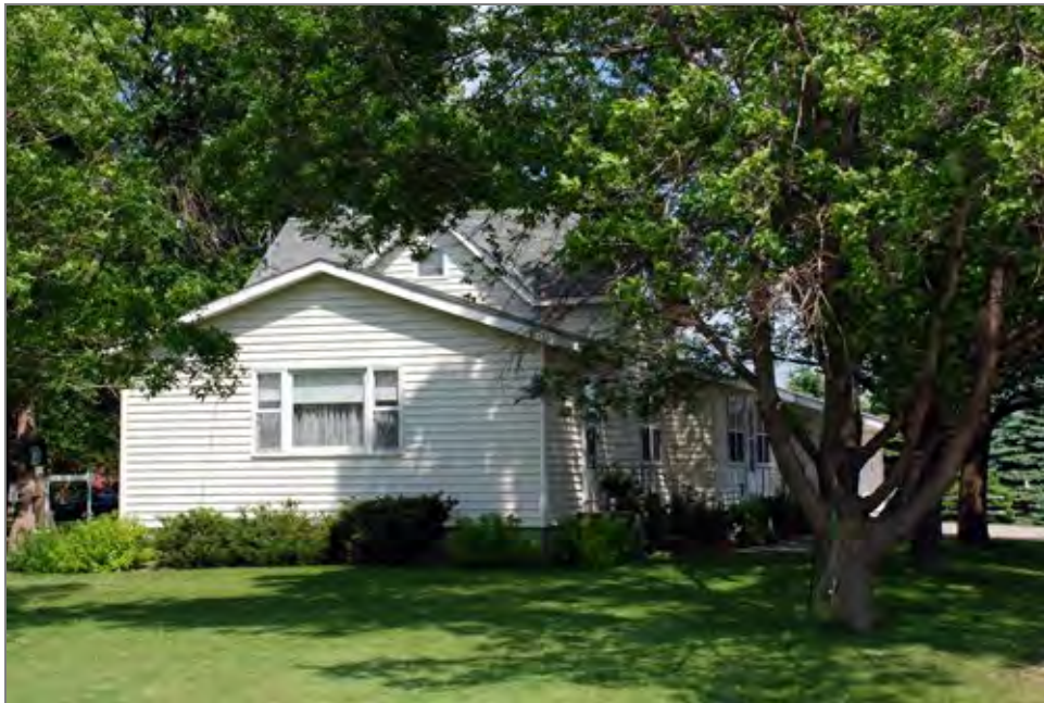
Field No. 73, House, facing NE
