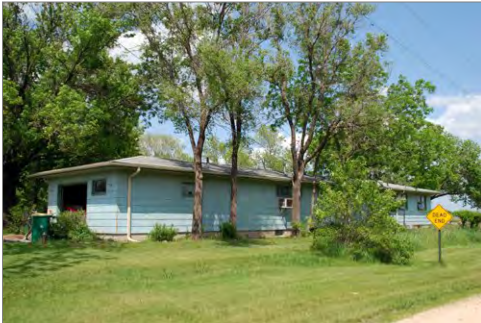
Field No. 69, House, facing NE
