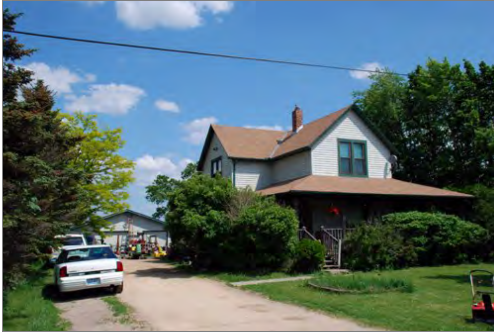
Field No. 70, House and Garage, facing E
