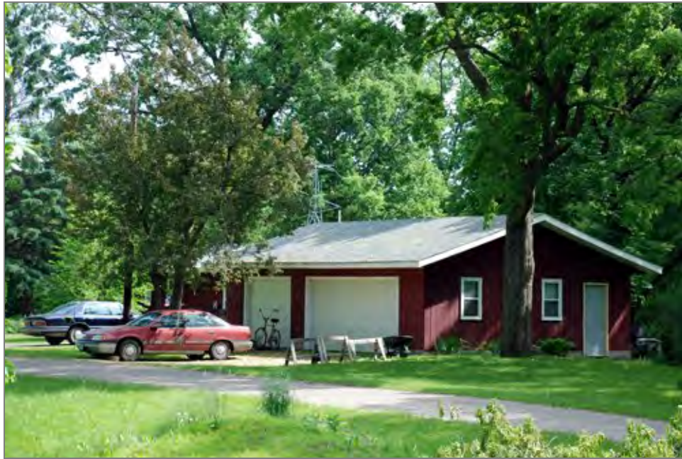
Field No. 7, House and Garage, facing NE
