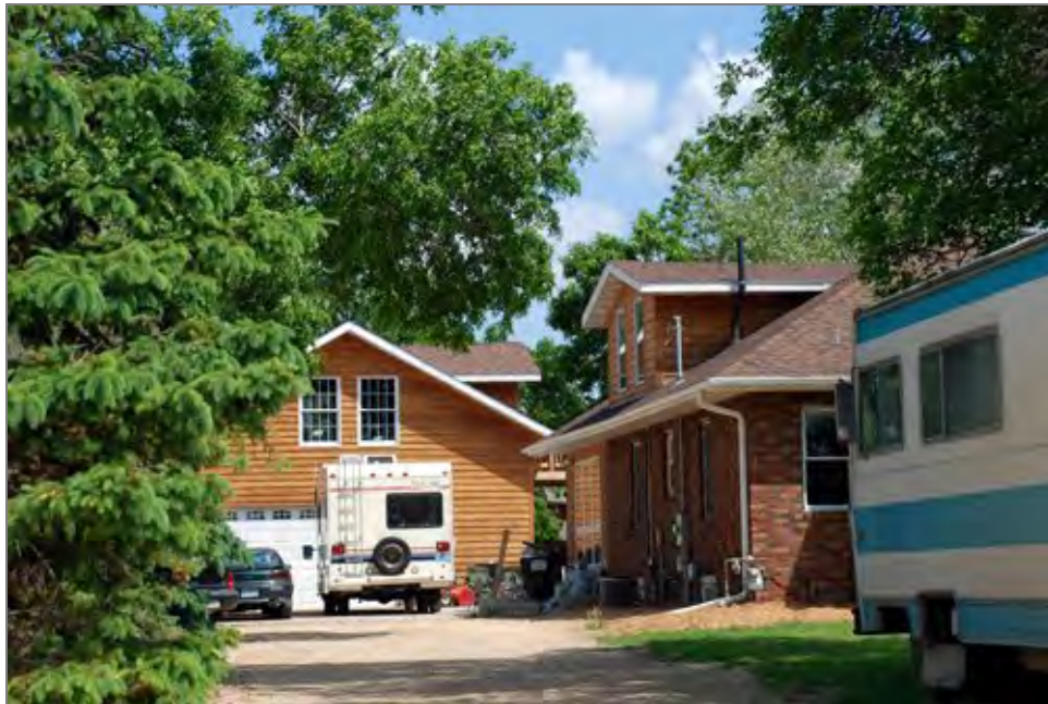
Field No. 65, House and Garage, facing E
