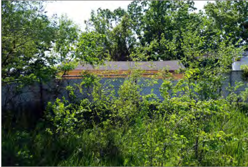
Field No. 92, House and Outbuildings, facing W
