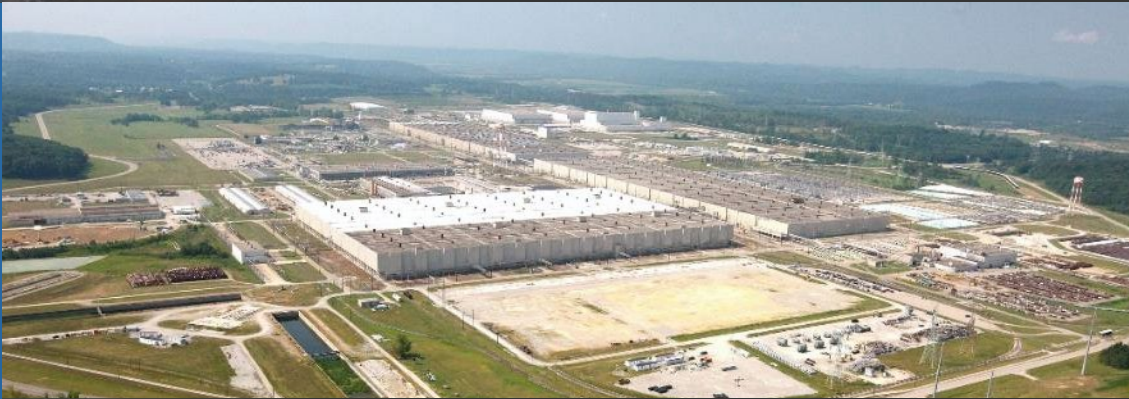
Portsmouth Gaseous Diffusion Plant
