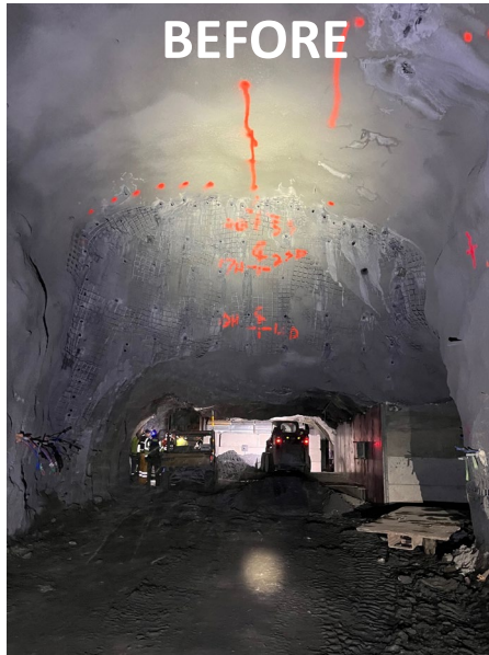
Adjusted “brow” to allow long materials to be maneuvered out of the shaft
