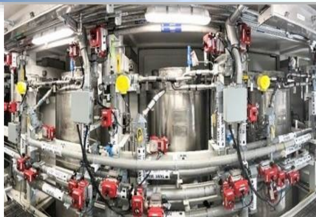
Tank-Side Cesium Removal System (Hanford)
