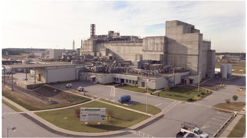
Defense Waste Processing Facility at SRS
