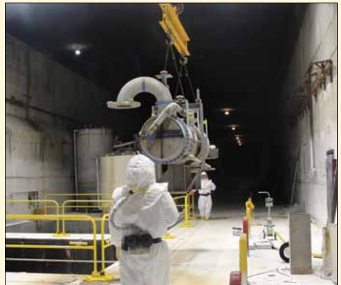
A heater is loaded into an open cell at U Canyon as work progresses to clear the deck of the facility.
