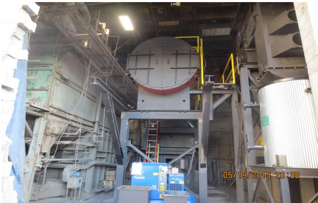
Figure 4 – Install New Boiler
