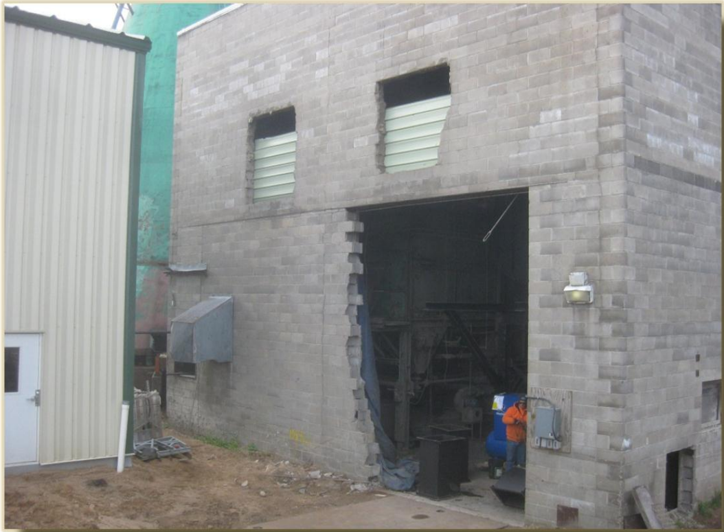
Figure 3 – Demo Old Boiler
