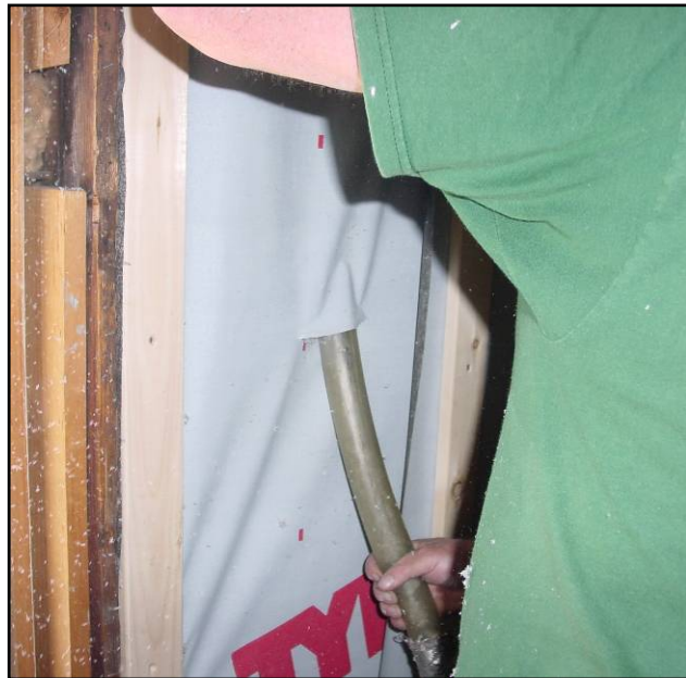
Dense packing the back of a knee wall with cellulose
