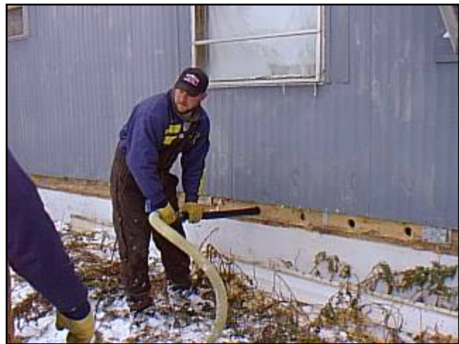
Blowing a mobile home floor
