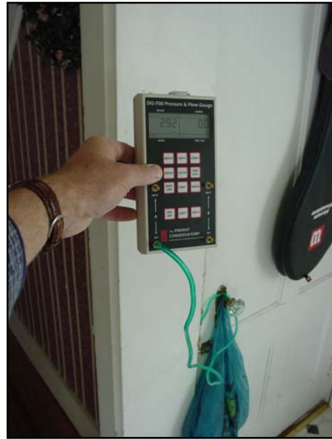
Zone pressure test to basement with blower door depressurizing house to -50 Pascals
