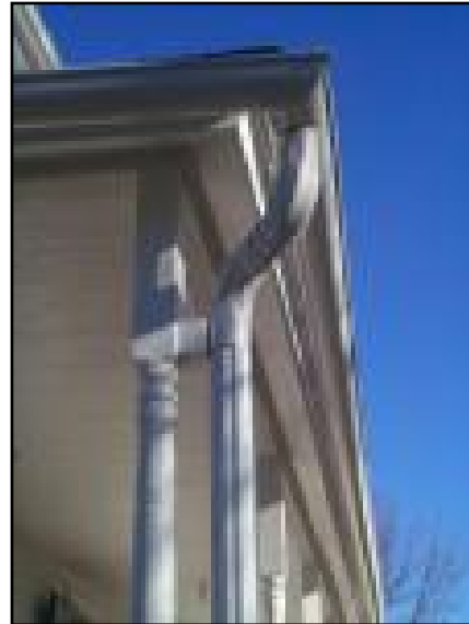
Gutter and downspout
