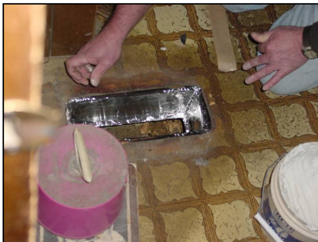
Using metal and mastic to seal mobile home duct boots
