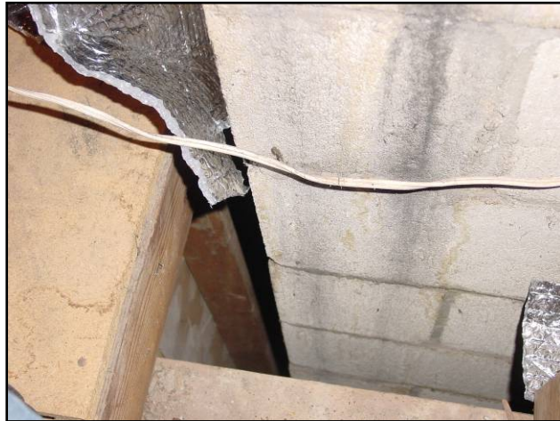
Foil faced bubble wrap may NOT be used for sealing chimney chases.
