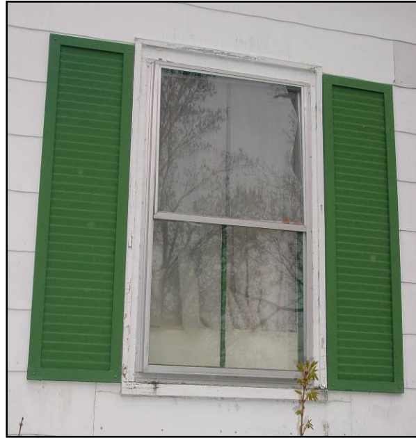
Double hung sash with exterior aluminum storm window
