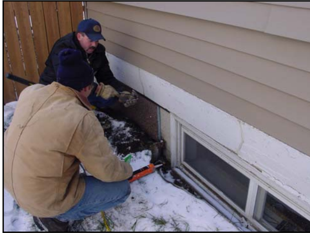
Installation of rigid exterior foundation insulation
