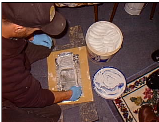
Sealing a register boot with duct mastic
