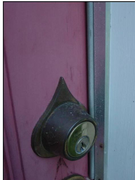
Exterior door metal/vinyl weatherstripping
