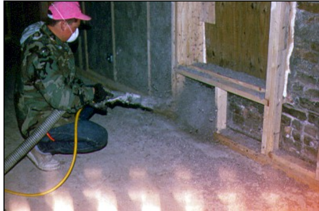
Wet spray cellulose being installed
