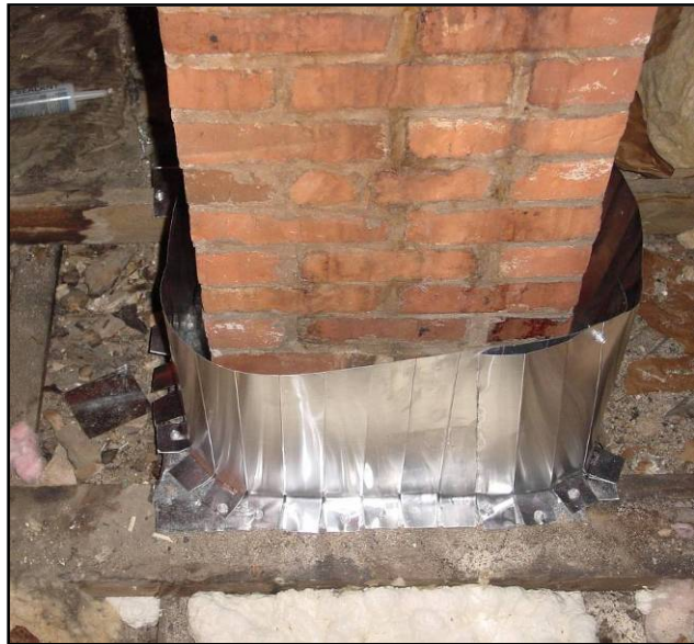
Chimneys must be blocked to keep cellulose at least two inches away from the masonry
