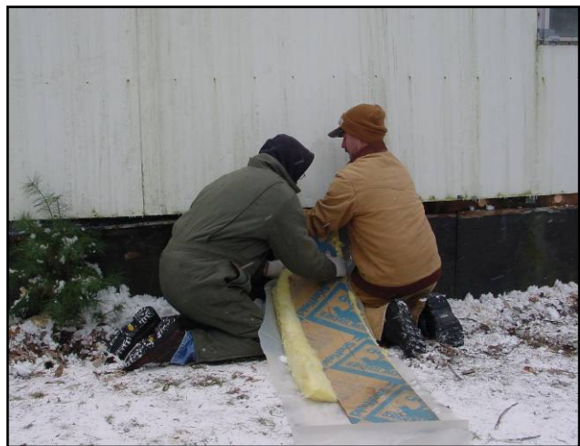
Batt-stuffing a mobile home wall cavity
