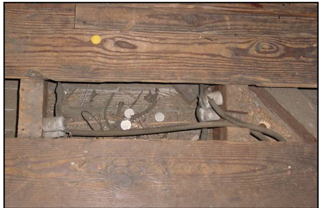
Knob-and-tube wiring can be hidden under attic floors; don't forget to inspect for it and then treat it accordingly
