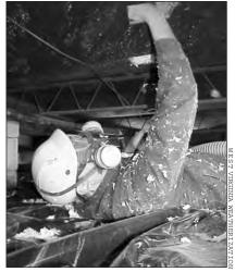
After cutting access holes through the belly board of the mobile home, push any existing insulation aside so that the flexible fill tube can slide the length of the joist cavity for a complete fill.
