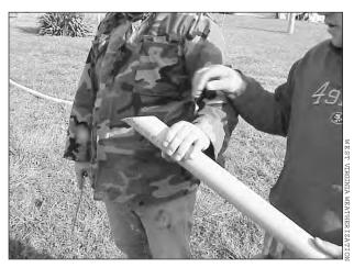
(left) After the duct is cleaned, fibered tape and mastic are used to air seal. A paint brush is the easiest ways to apply the mastic to the duct. (right) The end of the blow tube should be cut at an angle to help the tube slide over the existing insulation and past any obstructions in the cavity.
