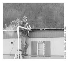
A worker blows fiberglass into the cavity of the mobile home roof. Note the  $2 \times 4s$  used as wedges to hold the roof cavity open. A small amount of blowback can be seen.
