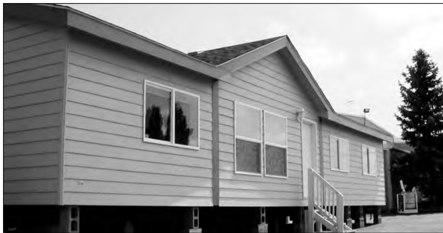
The Concept 2000 house was set up on the factory lot. Tests found the house among the tightest and stingiest ever built.
