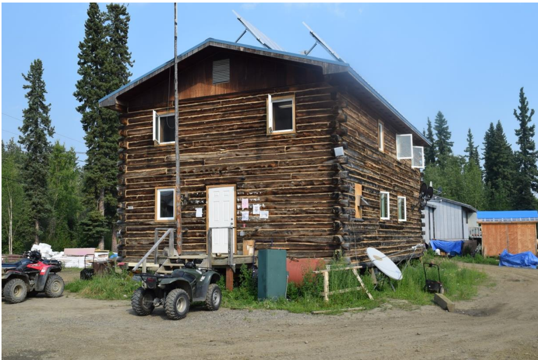
Figure 15 Koyukuk Office after renovations with new windows, new doors, and foundation.
