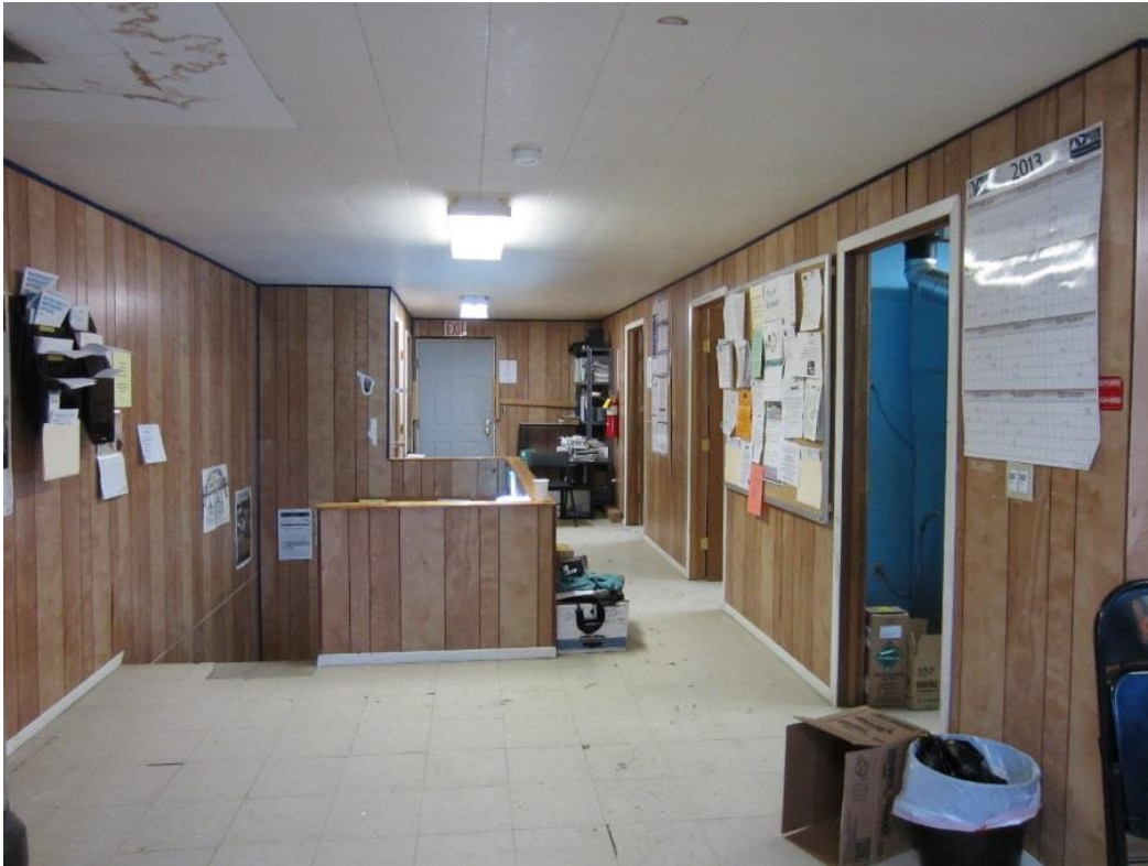
Figure 11 Koyukuk Upstairs before renovation
