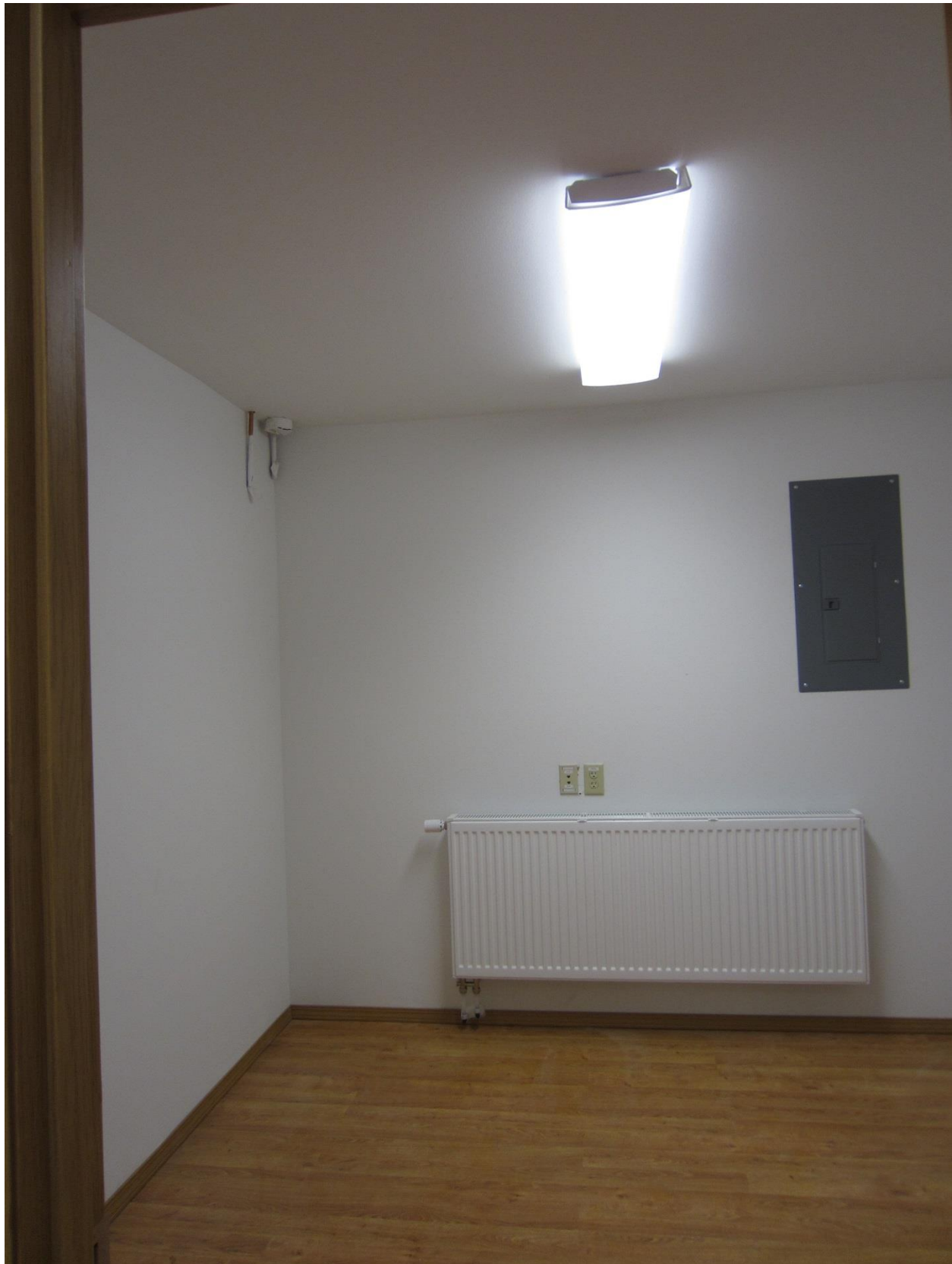
Figure 13 Koyukuk Office with new low temp register
