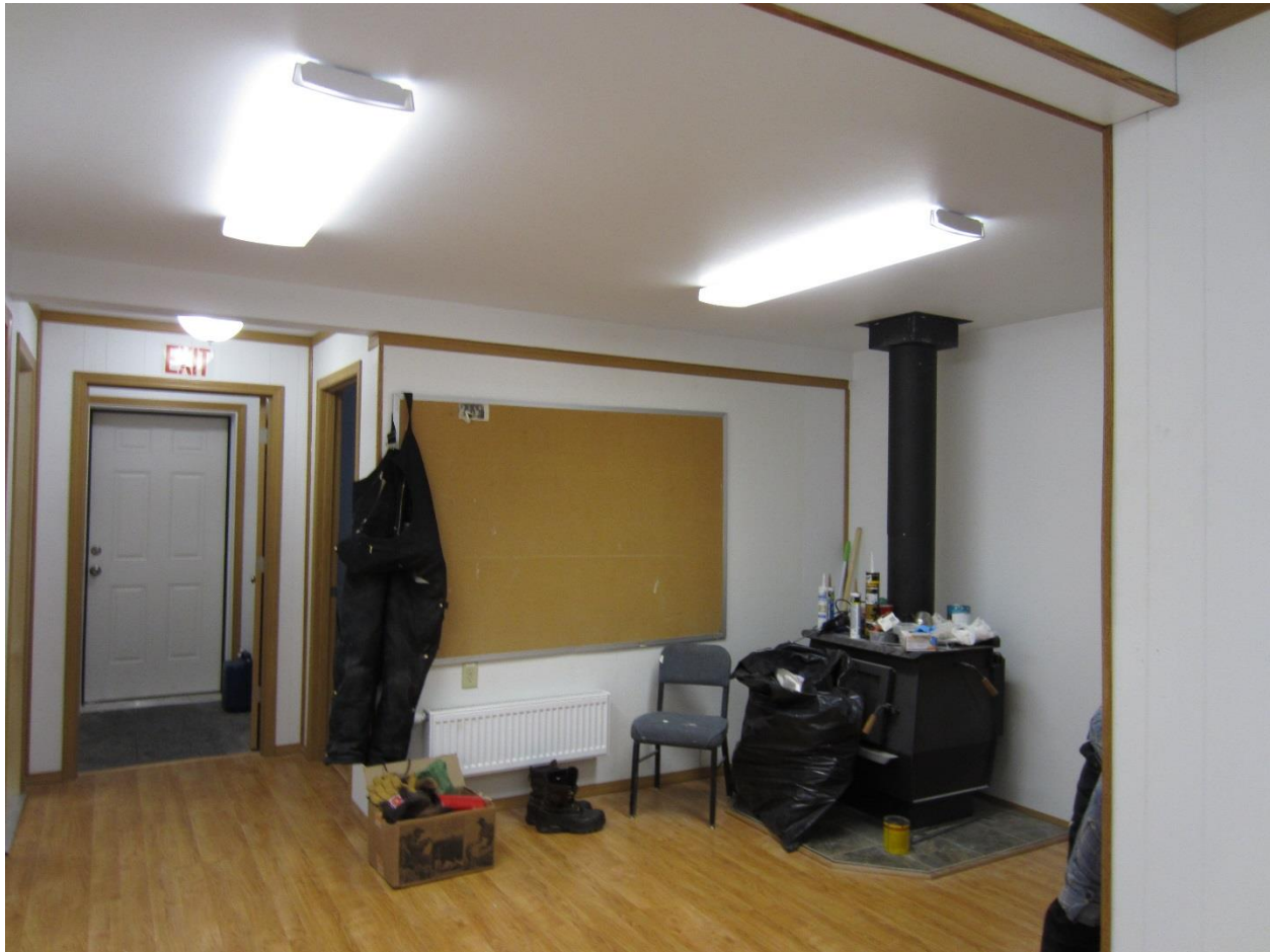
Figure 12 Koyukuk Entry area after renovation with new wood stove back up heat if generator breaks down and low temp register.
