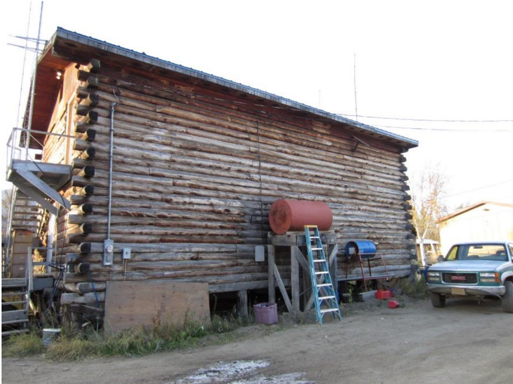
Figure 8 Koyukuk Office before renovation
