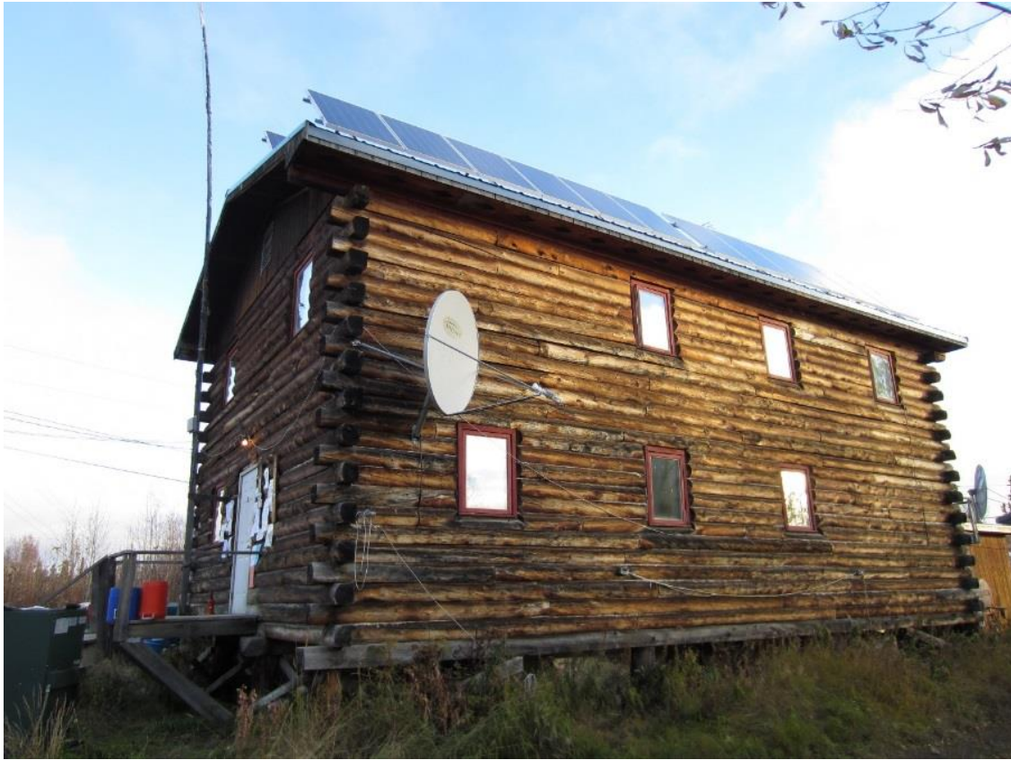
Figure 9 Koyukuk Office before renovations with old windows, old door and foundation.
