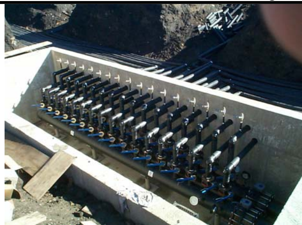
Cast Header Vault - Installation
