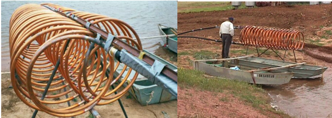
Figure 2.1. A 5-ton copper coil pond loop being installed in a pond.
