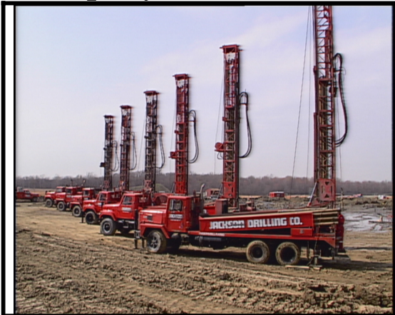
Large project drilling capability
