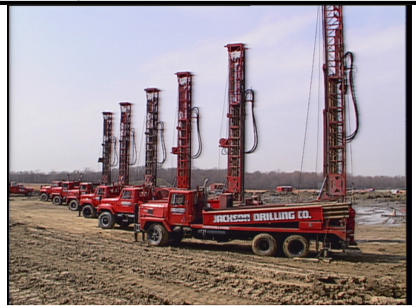
Geothermal Drill Rigs
