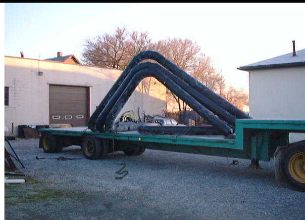
Large Pipe Fabrication
