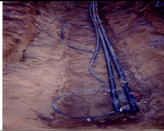
Pipe / Borehole Headering
