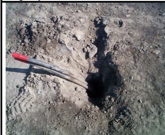
Borehole heat exchanger completion – grouting, spacing
