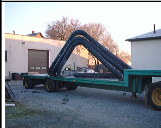
Fabrication of Large Pipe Fabrication
