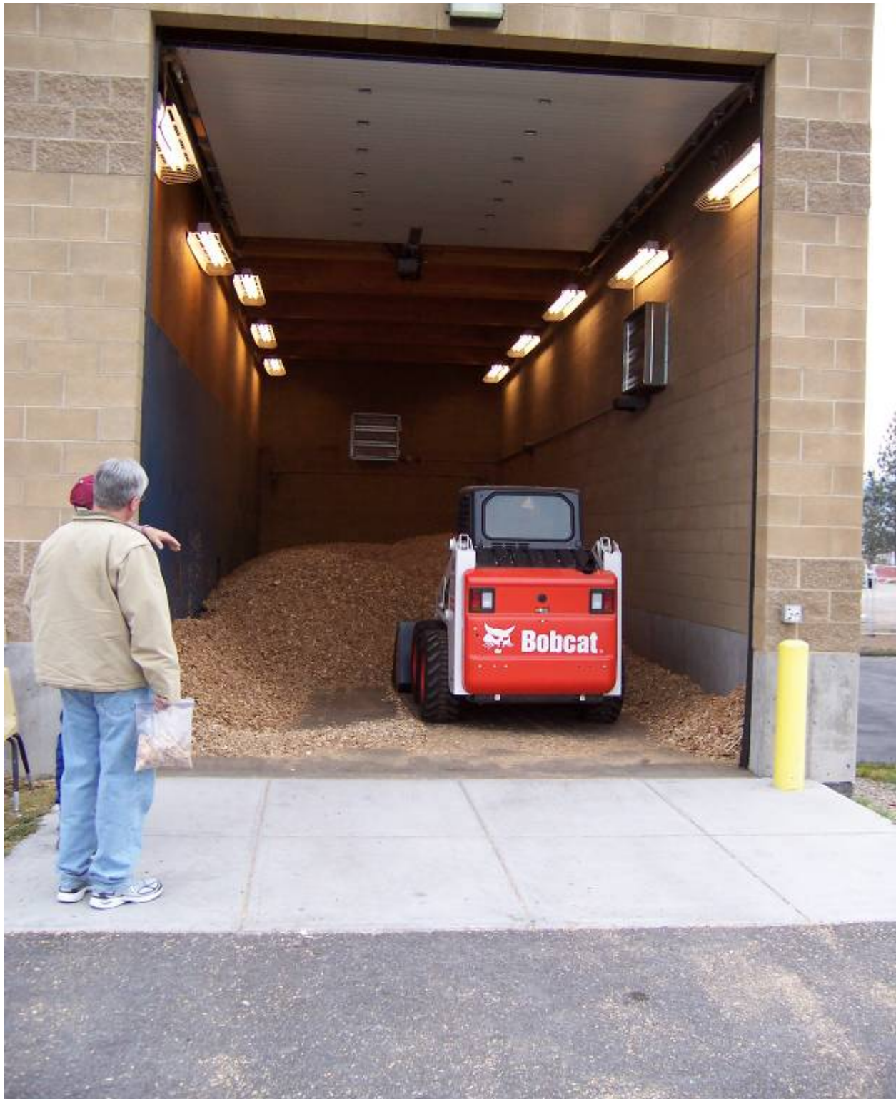
Victor School Biomass Operations Storage
