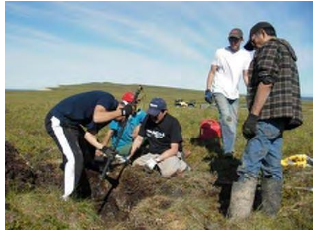
Installing plate anchors; D. Vaught photo
