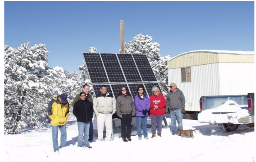
New NTUA Off-Grid Photovoltaic (PV) Hybrid Unit
