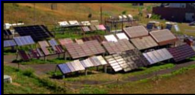
Outdoor Test Area
