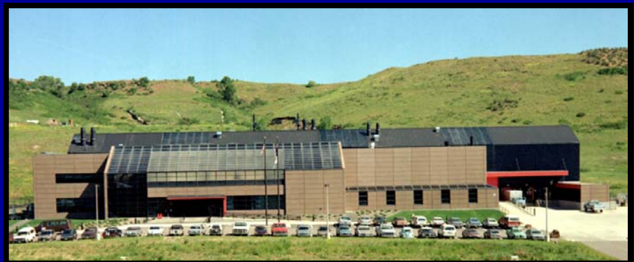
Field Test Laboratory Building (FTLB)
