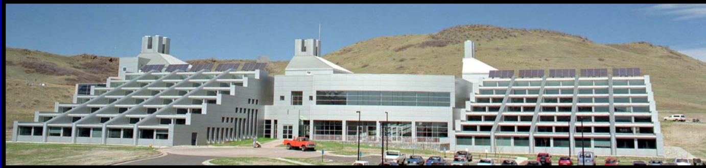
Solar Energy Research Facility (SERF)
