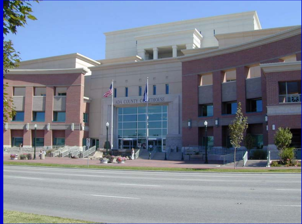
The Ada County Courthouse (Boise) uses the city geothermal district-heating system.
