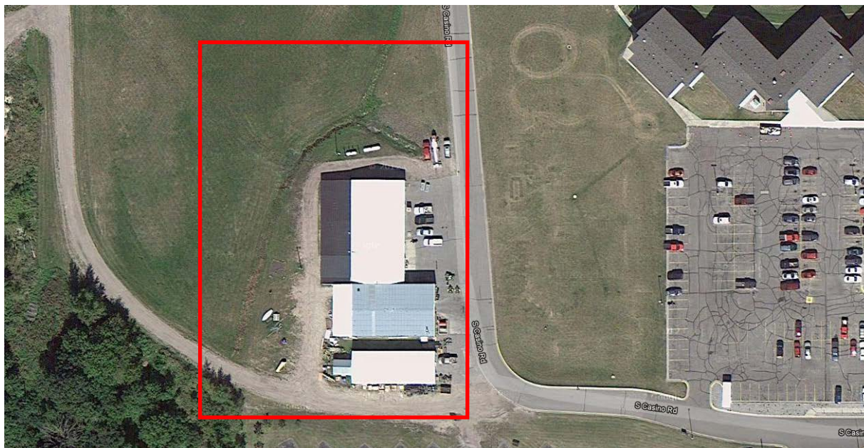
Figure 40. Mechanical and Maintenance Building Site
