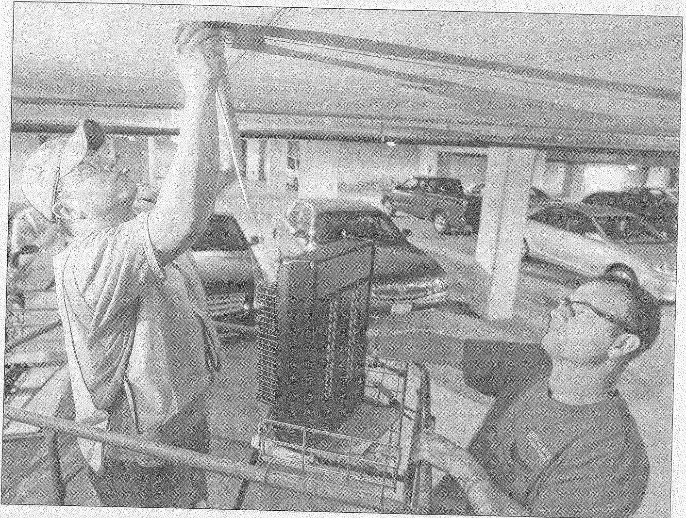
Apprentice electrician Brad Arreola (left) is aided by foreman Vince Mandella while installing an LED light Wednesday at Potawatomi Bingo Casino. The casino is having its parking garage lights replaced with LED fixtures that use less energy and have lower maintenance costs.
