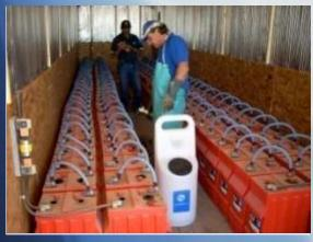
2 100Kw solar -diesel hybrid non-grid tied systems with 16kW solar- and 5400amp hour battery banks. Latest SatCon digitally integrated Inverters 50% -70% reduction in generator run time.
