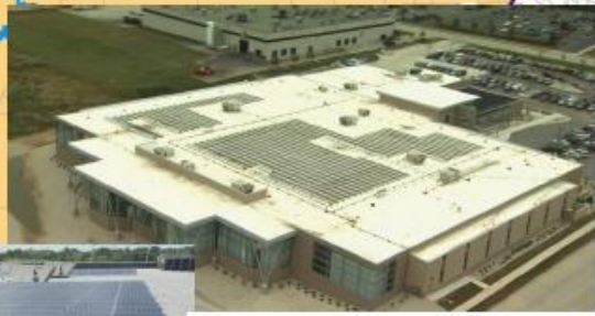
Example of facility solar electric in Wisconsin.
