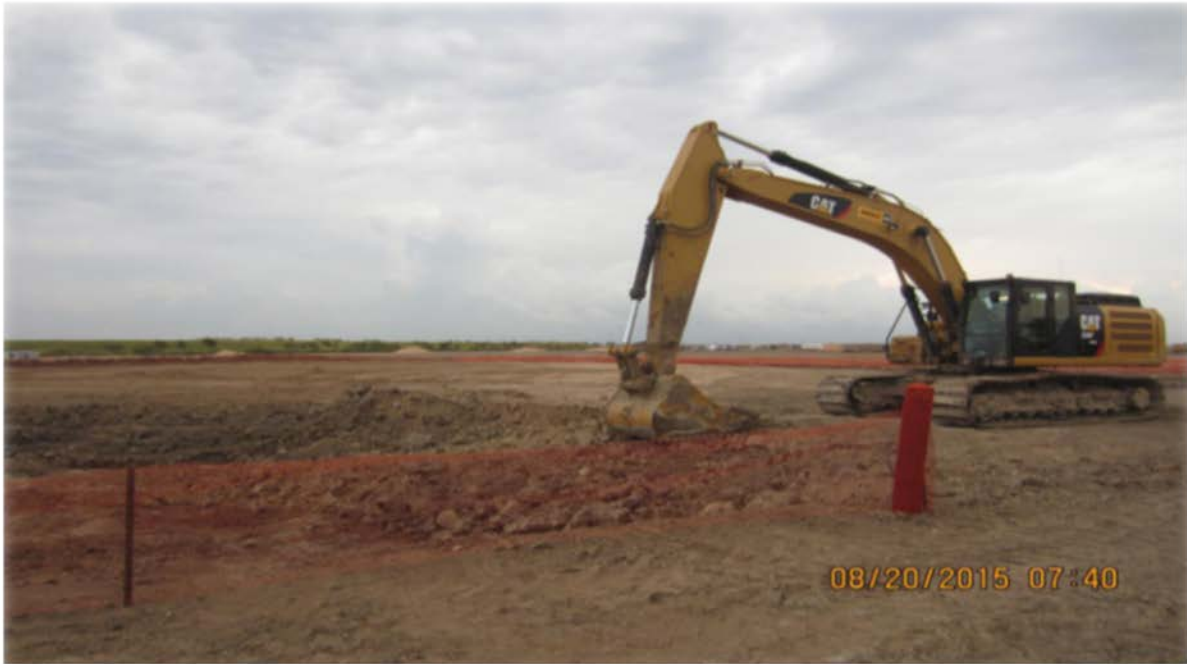
Tank A excavation – Bechtel
