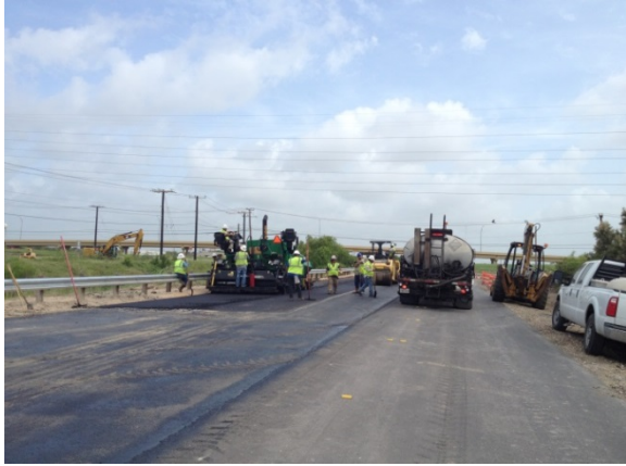
Paving of La Quinta Rd entry.
