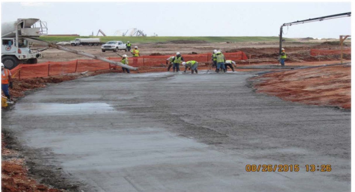
Tank A Mudmat– Bechtel
