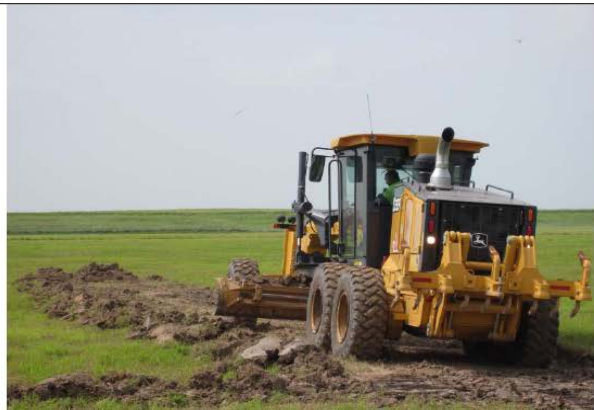
Clearing and Grubbing - Train 1, Priority 2 Area
