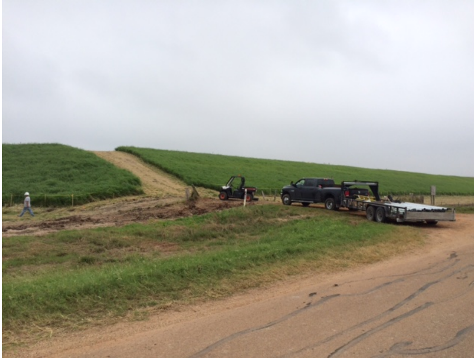
Photo 1. Installing fencing around Bed 22.
