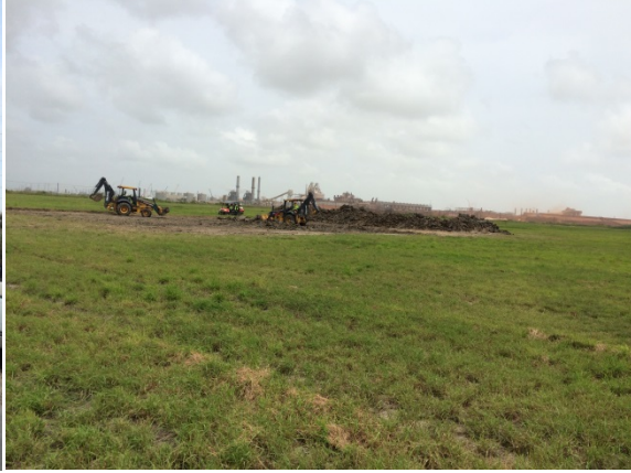
Excavation on train three for compaction testing.
