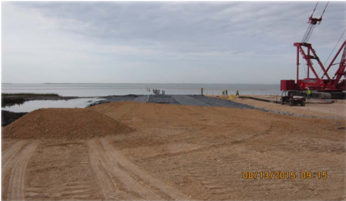
Construction dock area – Bechtel
