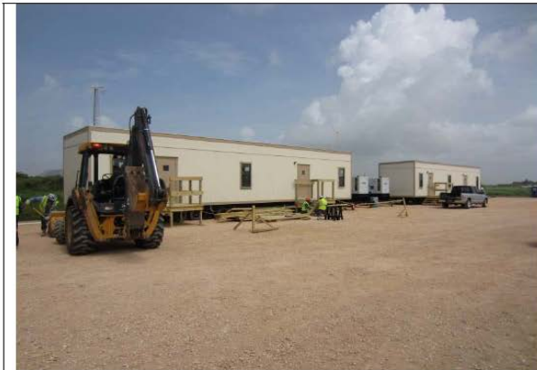
Installation of Pioneer Trailers Landings and Steps
