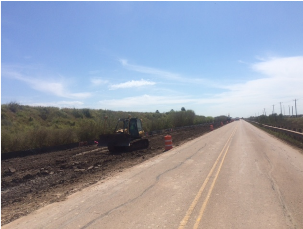
Photo 2. Widening La Quinta Road.
