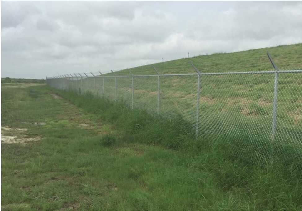
Photo 1. Installing fencing around Bed 22.
