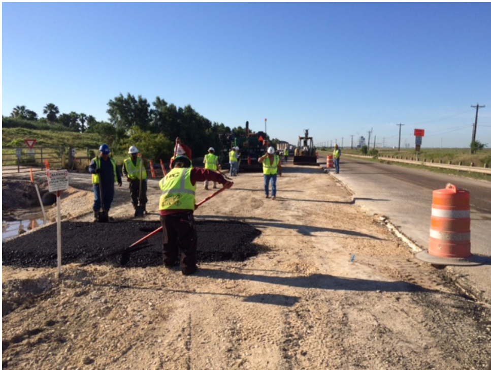
Photo 2. Widening La Quinta Road.
