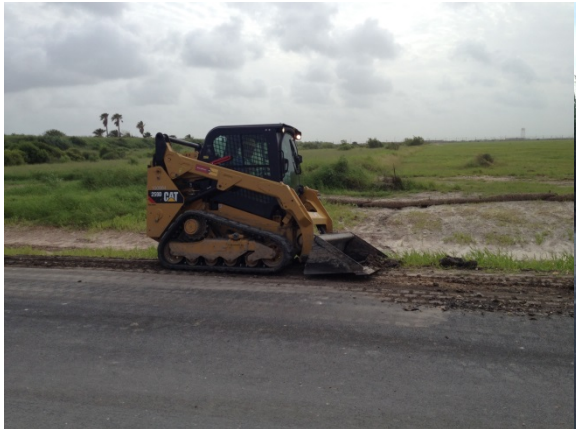
Grading ditches.
