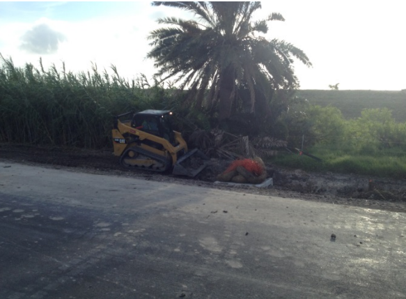
Grading east ditch on La Quinta Rd.
