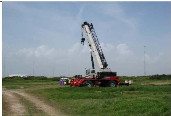
Marine Crane Mobilization and Installation – Priority 6
