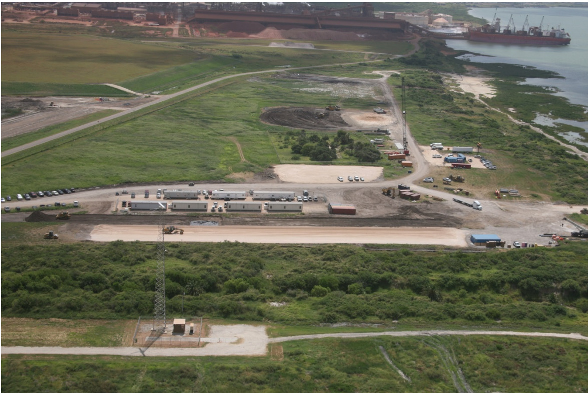
Shows the location of both Cheniere and Bechtel construction trailers.
