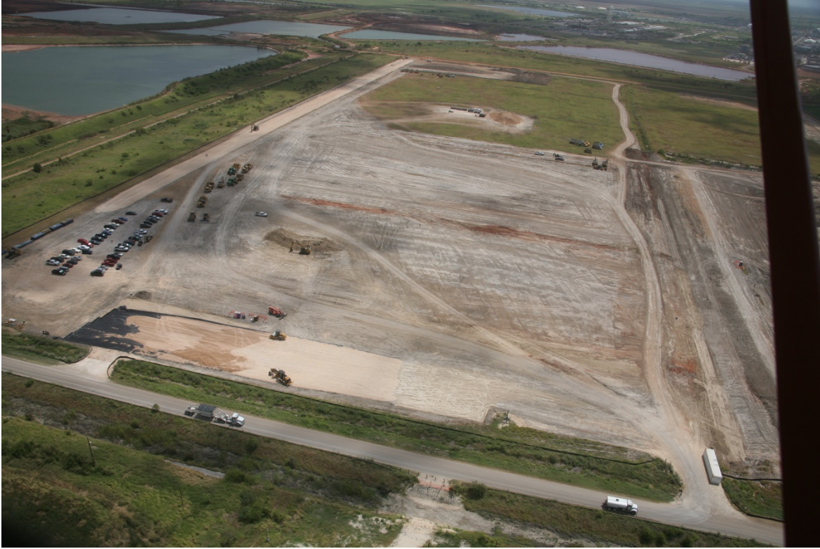
Indicates clearing and grubbing for the train area is well underway.
