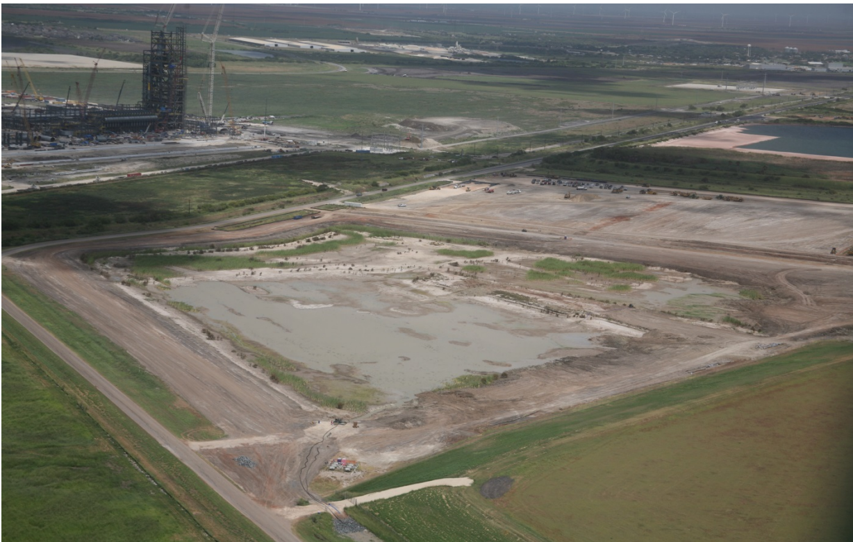
Aerial view of Bed 24 and ISBL site
