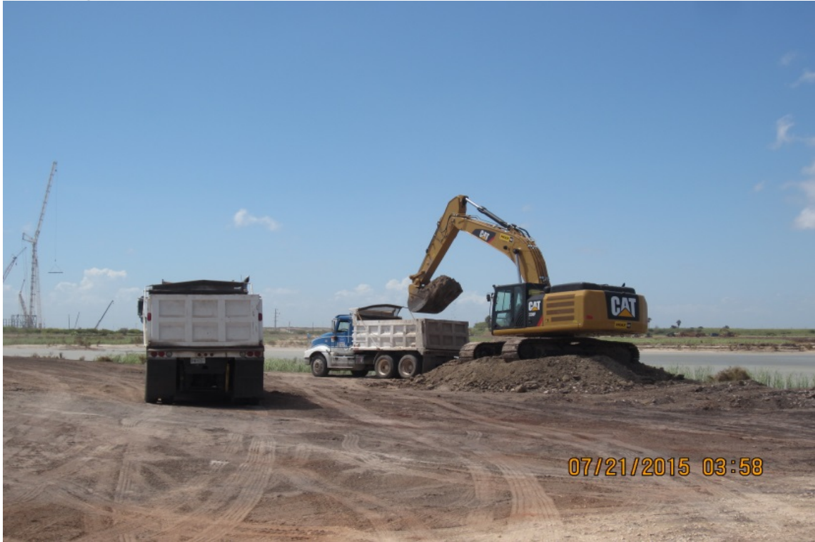
Excavation BED 24 – Bechtel
