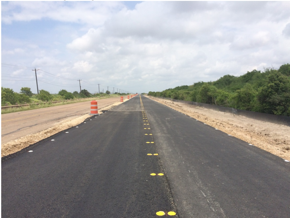
Photo 2. Widening La Quinta Road.
