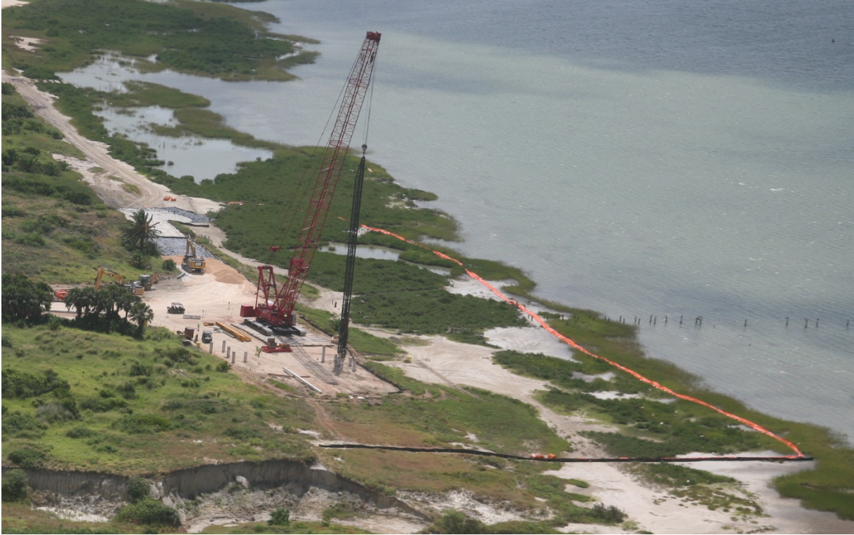
Installation of test piles
