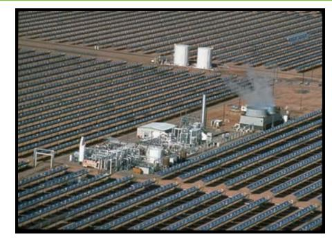
Total reflective area > 2.3 Mill. m<sup>2</sup> More than 117,000 HCEs 30 MW increment based on regulated power block size
