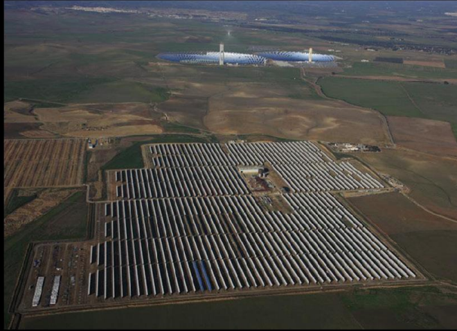
Abengoa 50MW Trough Plants Seville, Spain
