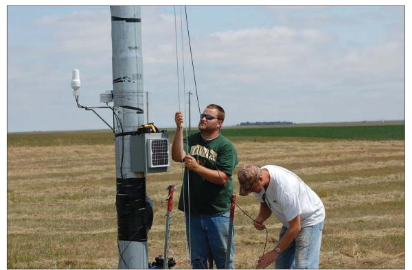
Photo 1. WPC and ETC staff raising 45m microphone on MET tower
