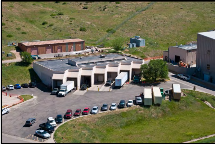
Shipping and Receiving Facility
