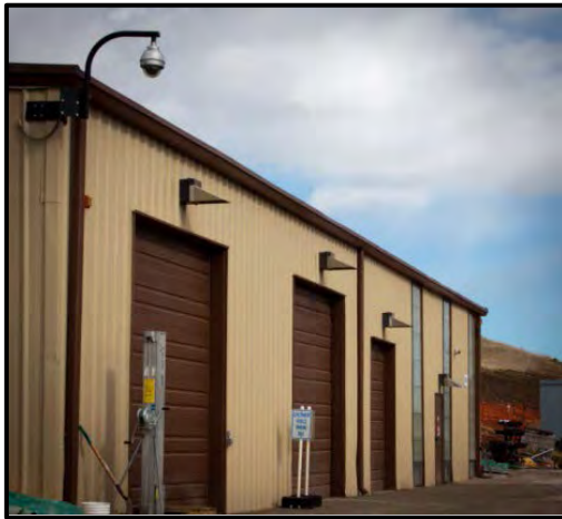
Facility Maintenance Building
