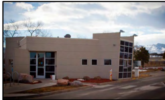
Site Entrance Building
