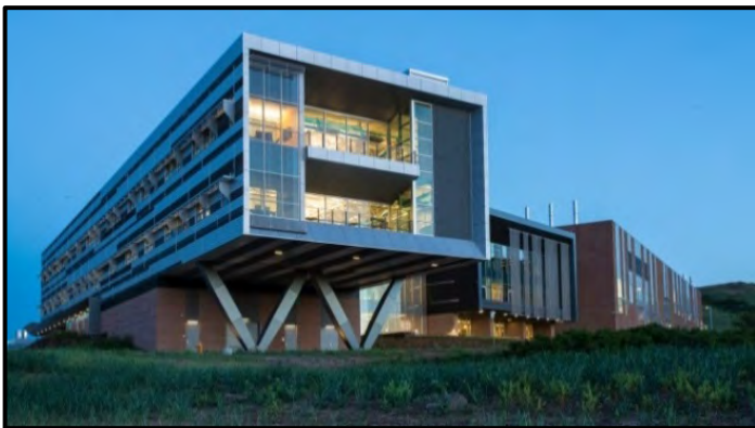
Energy Systems Integration Facility
