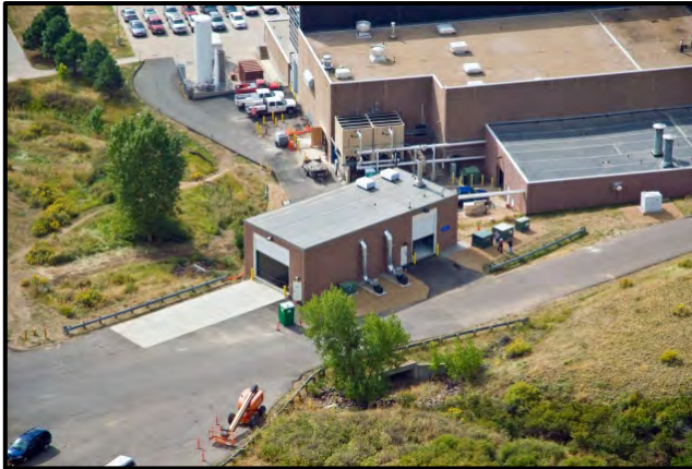
Renewable Fuel Heat Plant
