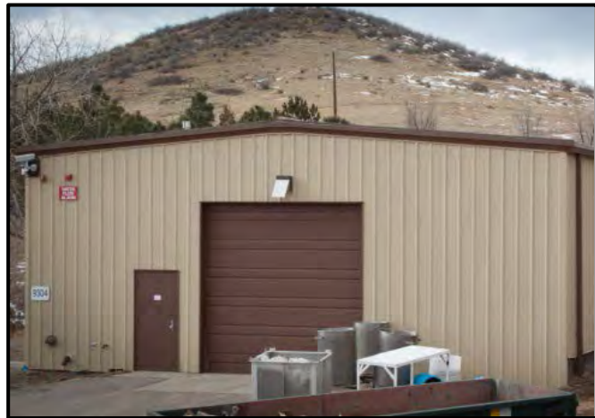
Bulk Storage Building
