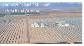
280 MW Solana Parabolic Trough Plant with 6 hours storage, Gila Bend, AZ
