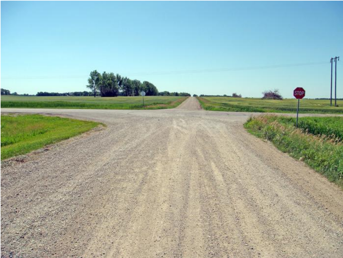
Normal road condition at Intersection 59 th Avenue and Highway 17.
