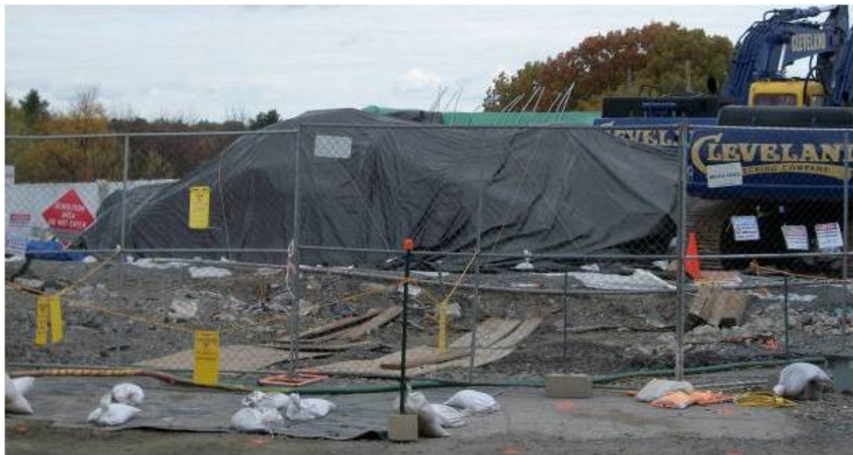
Figure 2-4: Building Footprint Taken Afternoon of October 23, 2010
