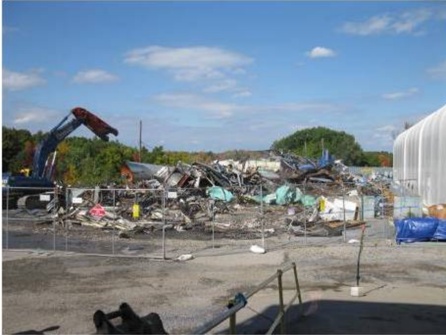
Figure 2-1: Facing North of the Building H2 on the Afternoon of September 25, 2010
