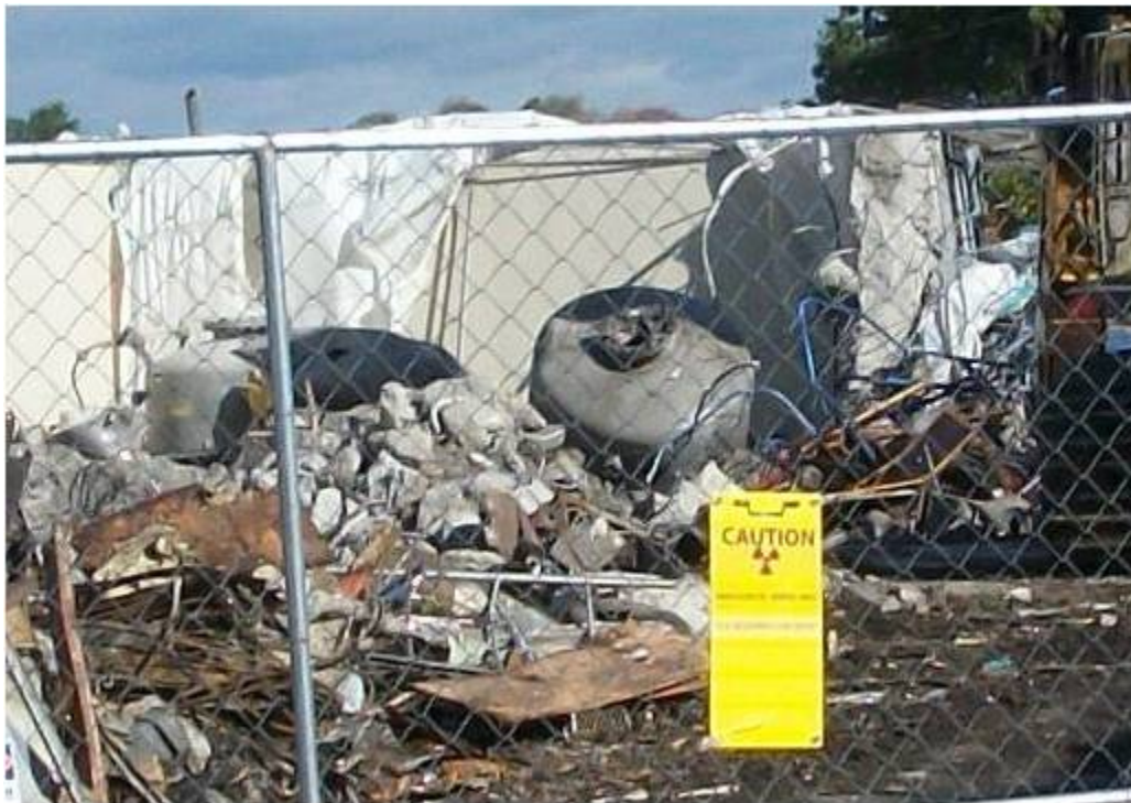
Figure 3-2: September 29, 2010 Post Column 113-A Removal
