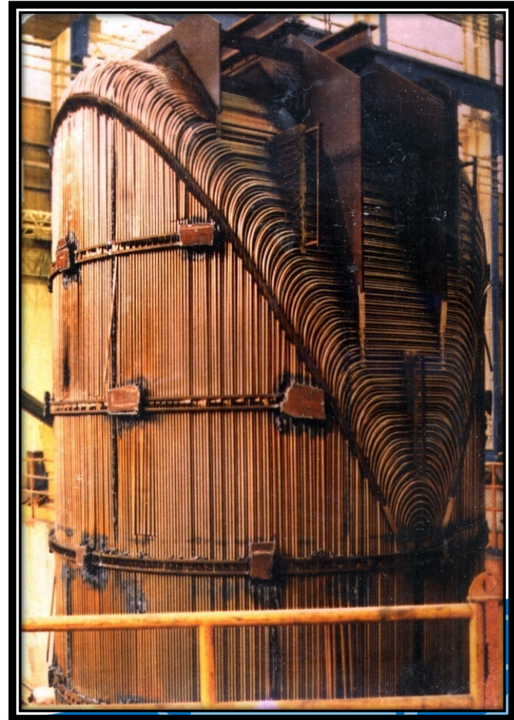
Example: Steam Generator Internals
